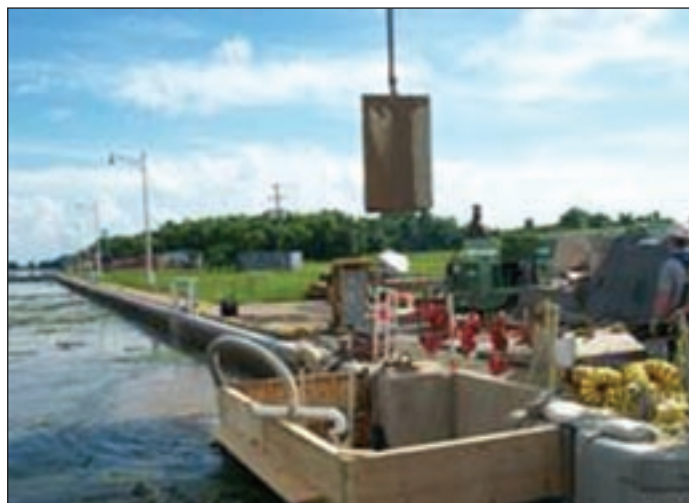
Crane lifts concrete block.
