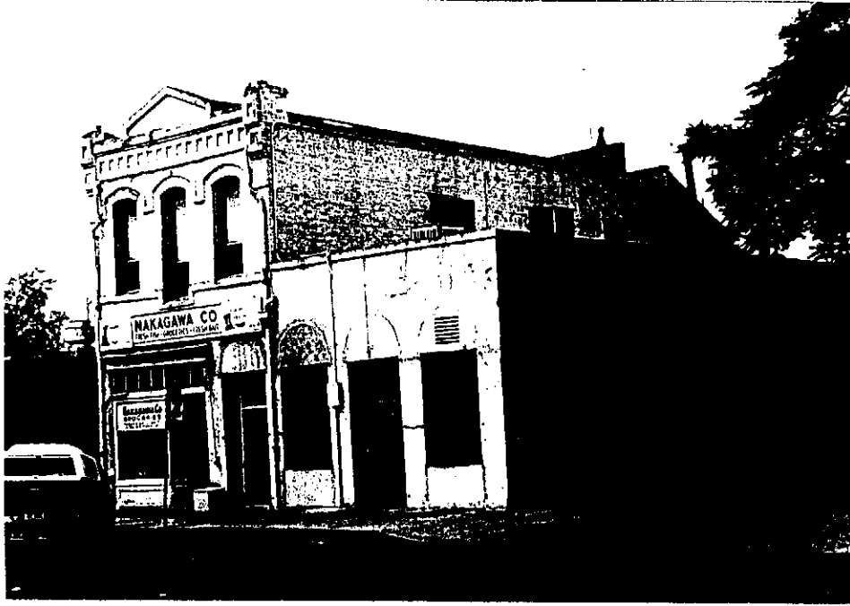
Photo No. 17 306 and 308 C Street, from northeast
