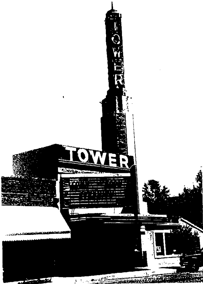
Photo No. 19 103 D Street, from northwest
