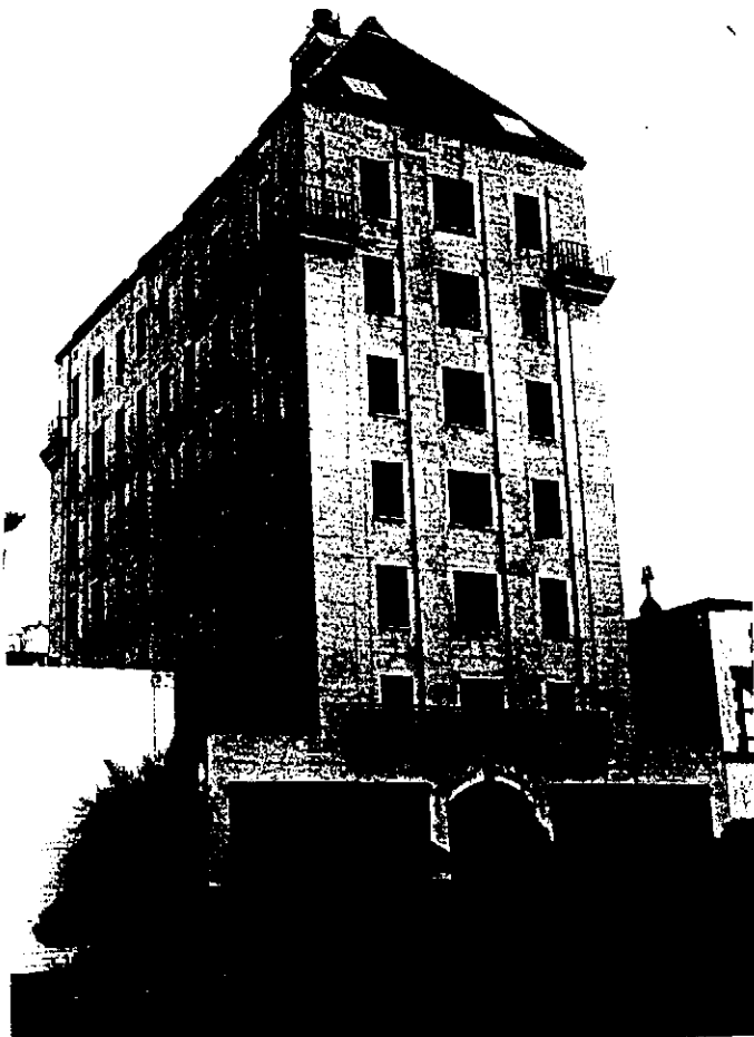
Photo No. 8 421-25 Fourth Street, from southwest
