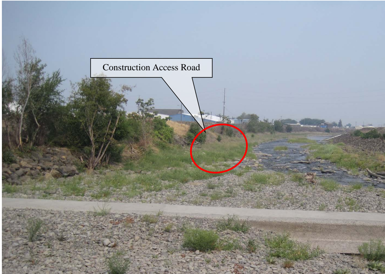
Photo 2-1. Potential Equipment Access from the Western Levee to the Drop Structure. The area within the blue outline is the approximate anticipated diversion and fill area if the thalweg remains against the levee. Note that the scale of the sketch and the photo are not accurate to the exact affected area and should not be interpreted as such.
