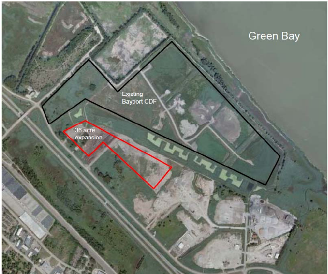
Figure 6. Future Expanded Dredged Material Placement Area at the Bayport CDF site.
