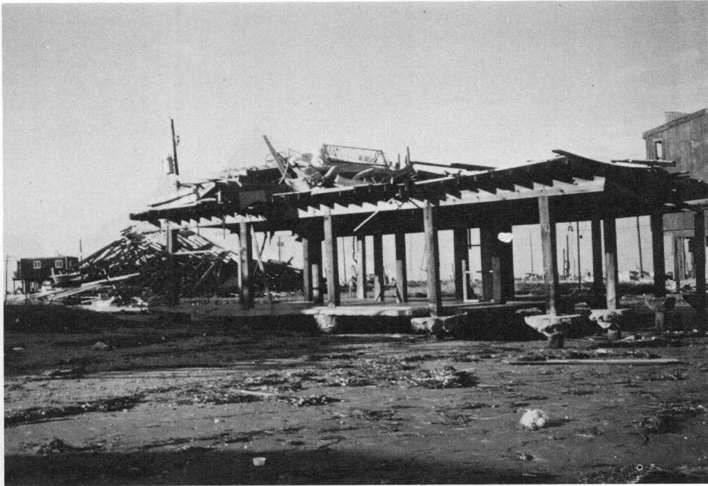
FIGURE 4.43 Example of a superstructure blown away by the wind. A mound of lumber, furniture, and appliances is in the backyard of the house.
