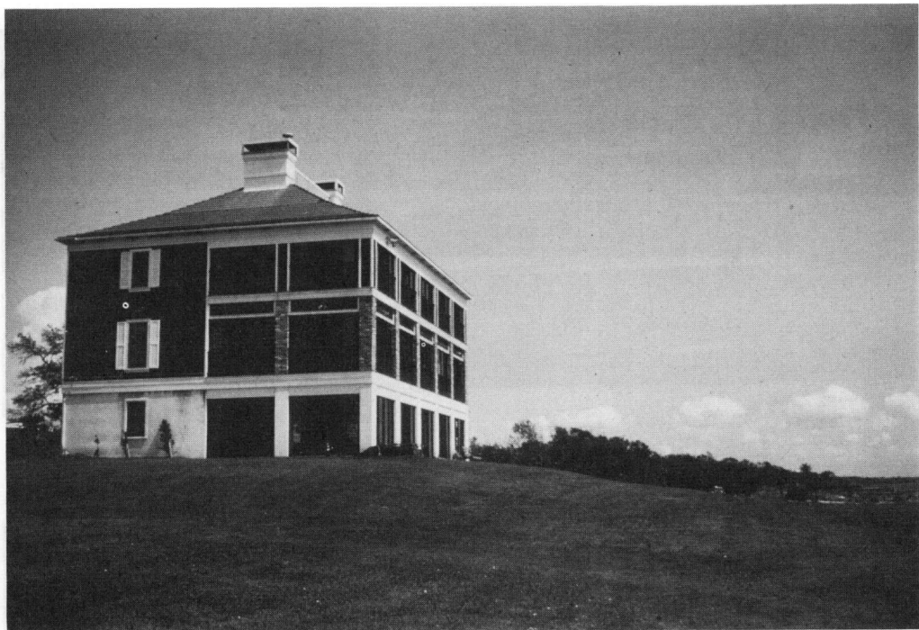
FIGURE 4.62 This mansion survived the storm very well.
