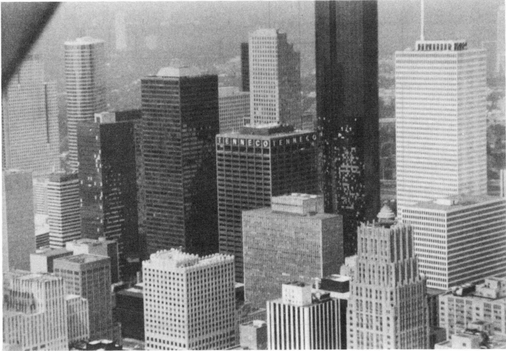
FIGURE 4.2 General view of the Houston central business district toward the west.
