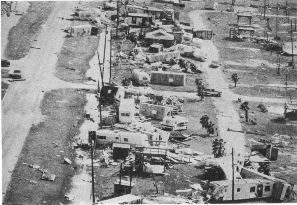
FIGURE 4.28 Damaged mobile home park on West Beach.
