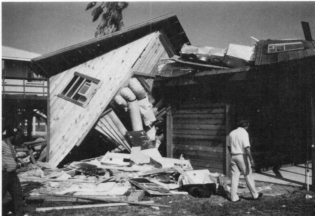
FIGURE 4.48 Typical example of poor connections between sub-systems.
