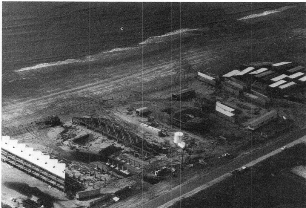
FIGURE 4.53 General view of a modular condominium project that experienced damage from wind and storm surge.
