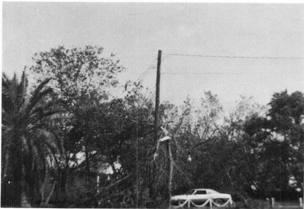
FIGURE 5.7 Typical failure of utility line caused by fallen trees in Seabrook.
