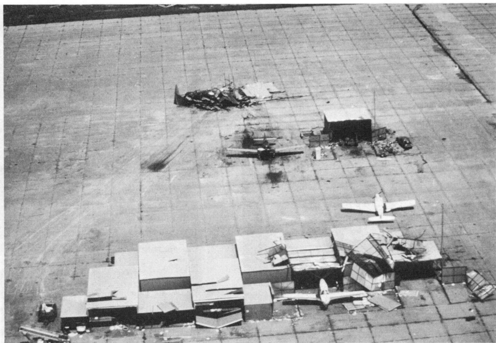
FIGURE 4.38 Damaged hangars and small aircraft at Galveston Airport.
