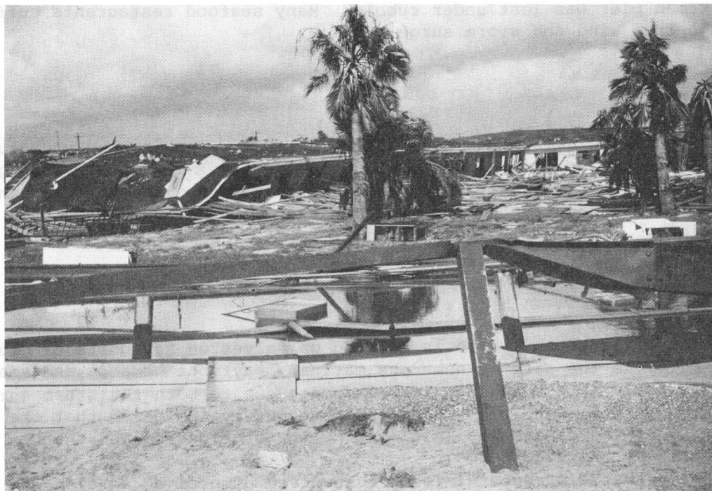
FIGURE 4.57 An elevated motel transported off its foundation by the storm surge.
