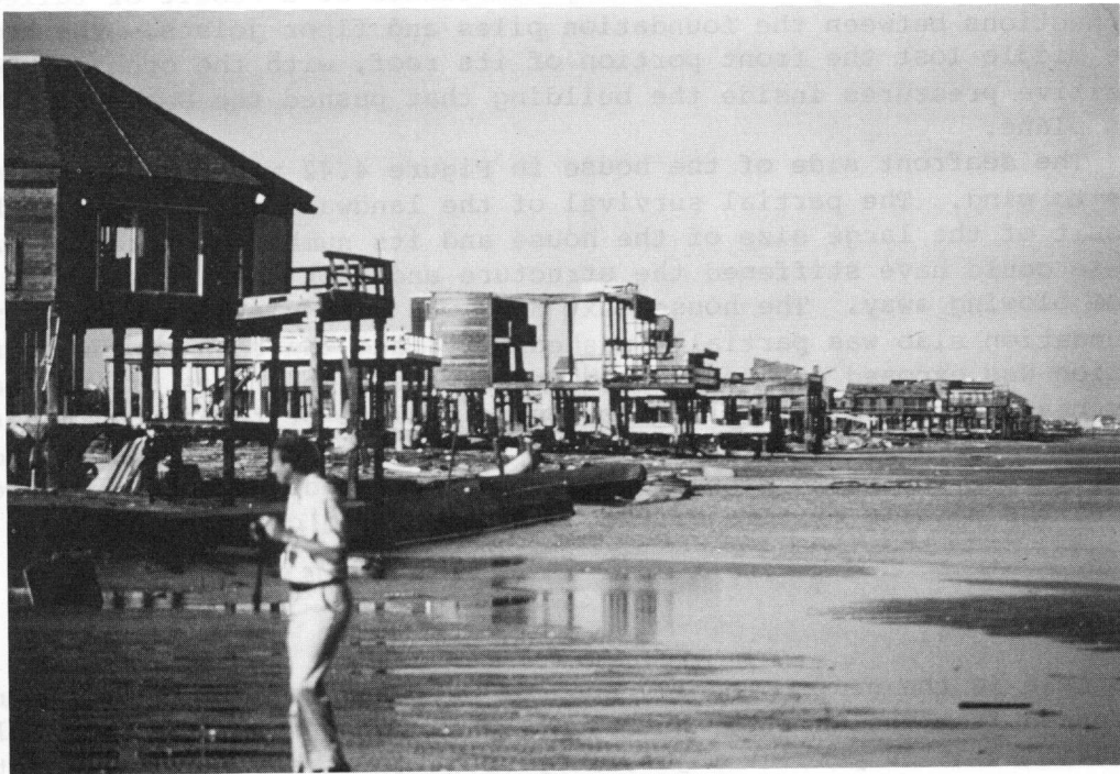
FIGURE 4.40 General view of damaged houses along Terramar Beach.
