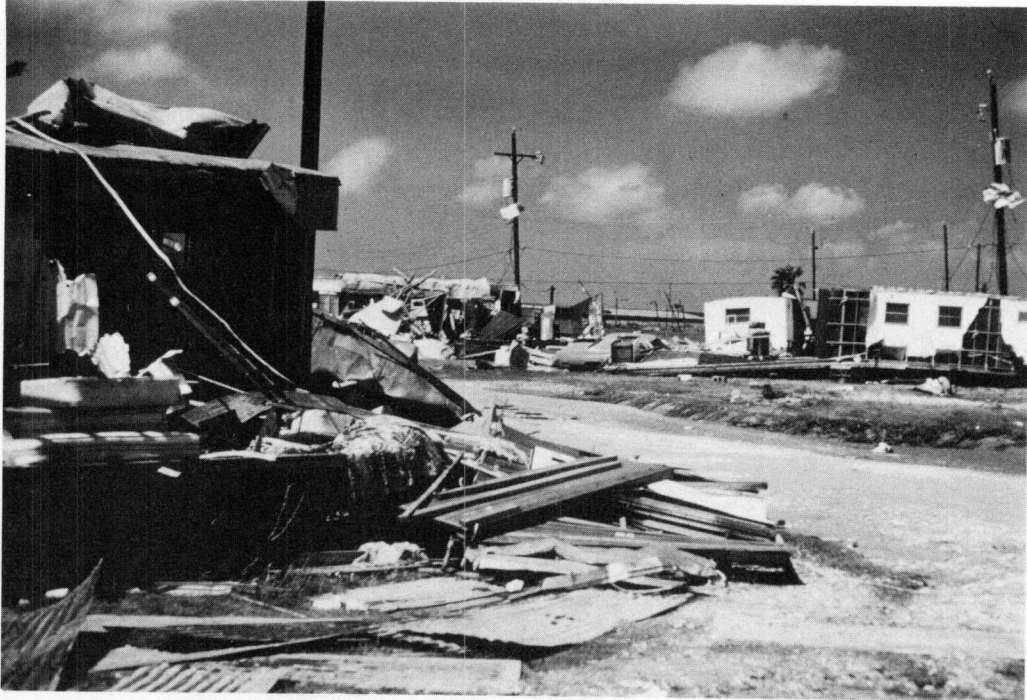
FIGURE 4.26 Damaged mobile home park on East Beach.
