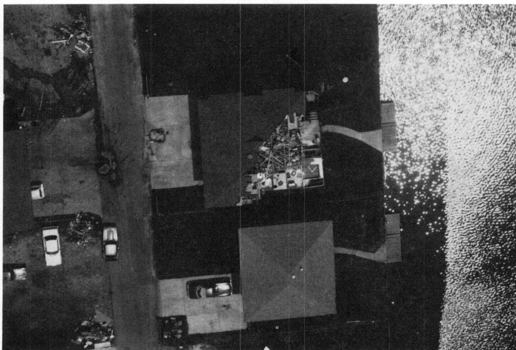
FIGURE 4.54 Aerial view of roof damage.
