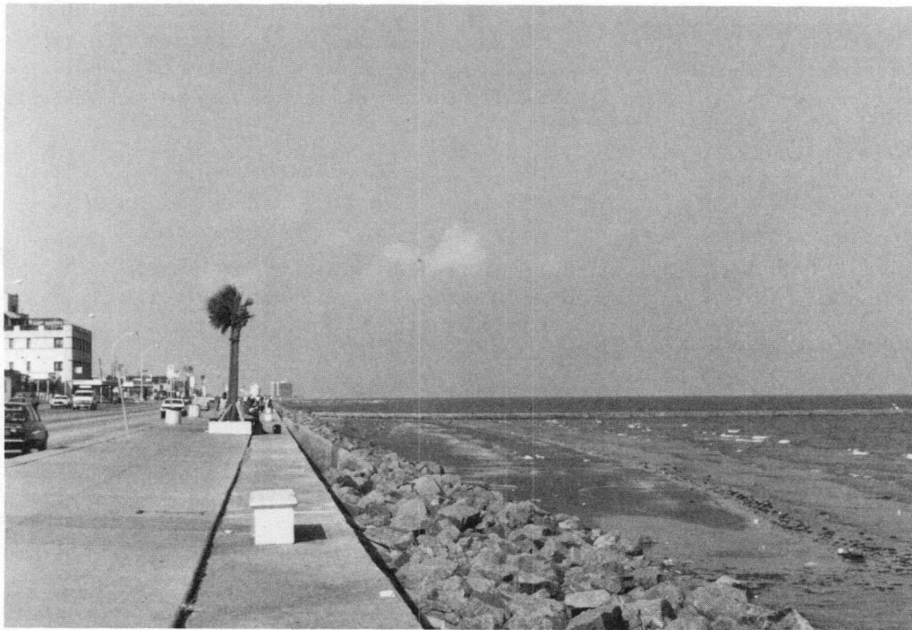
FIGURE 4.56 Galveston seawall and groin.
