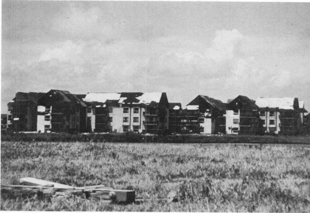
FIGURE 4.32 Roof damage to apartments near the seawall.
