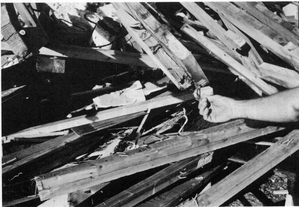
FIGURE 4.44 Details of toe nail connections.
