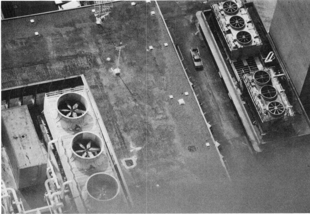
FIGURE 4.11 General view of the roof of the Tenneco Building.
