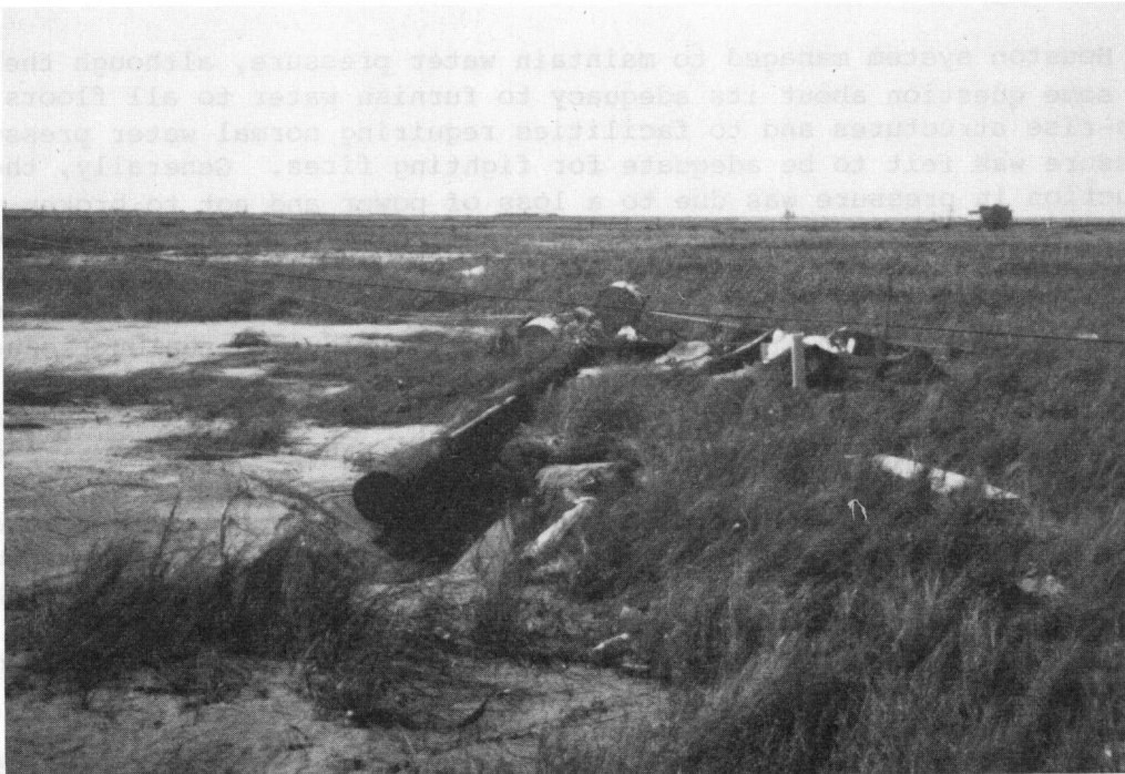
FIGURE 5.5 Typical failure of utility pole on East Beach, Galveston Island.
