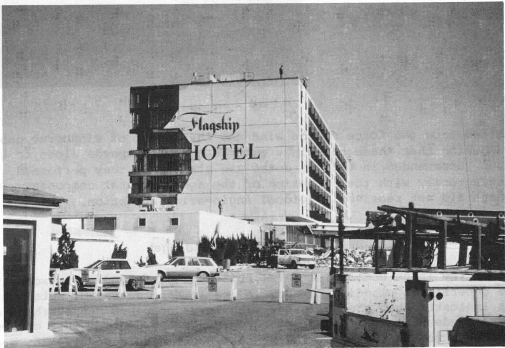
FIGURE 4.23 Damage to the facade of the Flagship Hotel.
