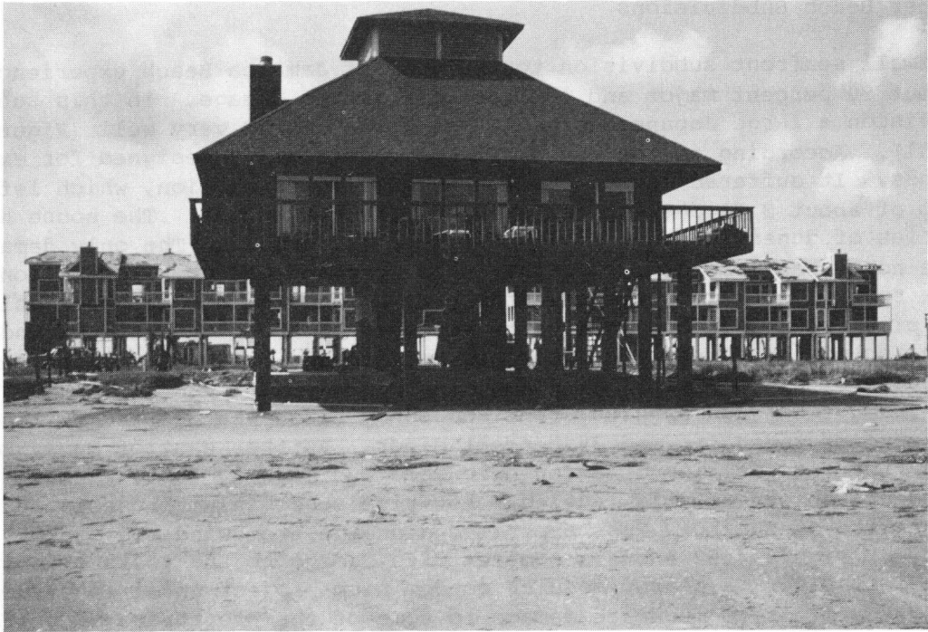
FIGURE 4.51 Example of a well-constructed house that performed very well except for erosion around the foundation.
