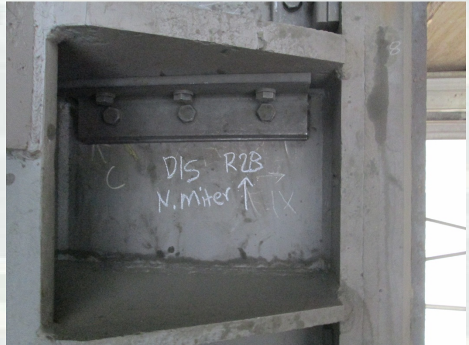
Bolted Angles Miter Block Crack Repairs
