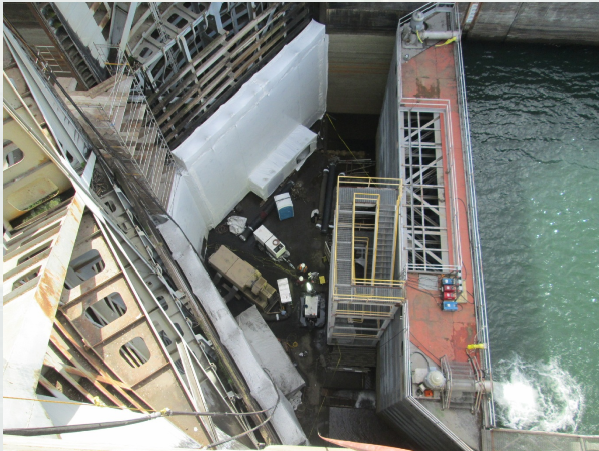
Coal Tar Removal Operations
