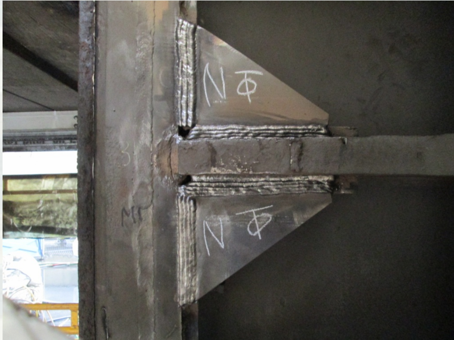
Welded Stiffening Brackets Miter Block Crack Repairs
