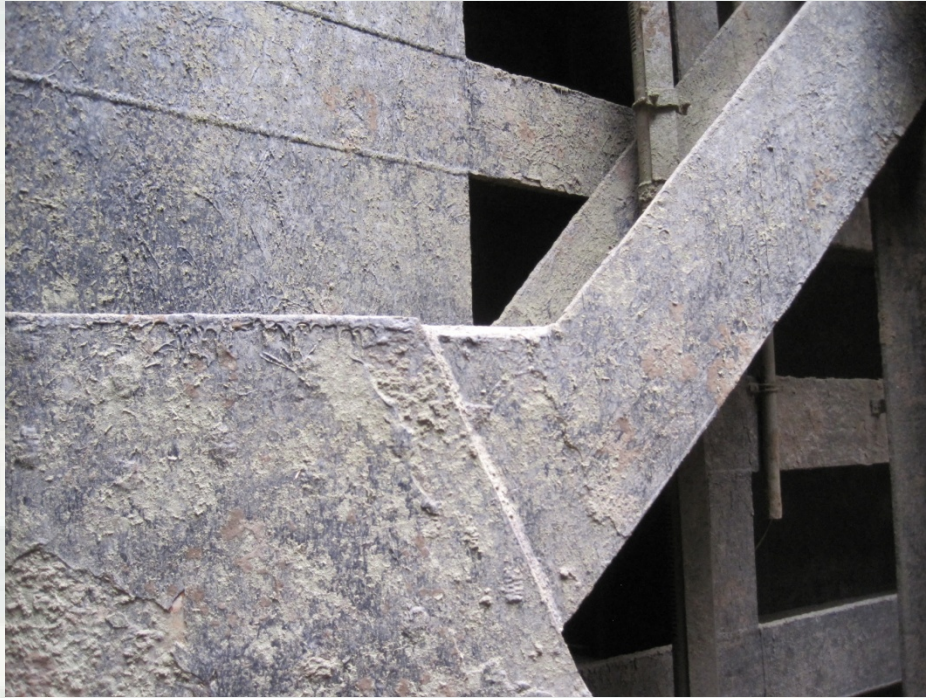
Coal tar coating on submerged areas of the gate structure
