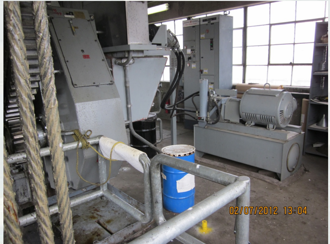
Existing Hydraulic Power Unit and Motor
