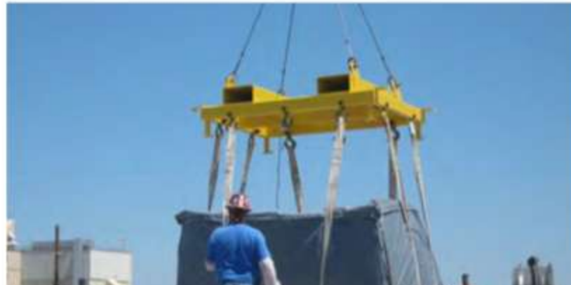
W.R. Grace Building 23 Remediation
