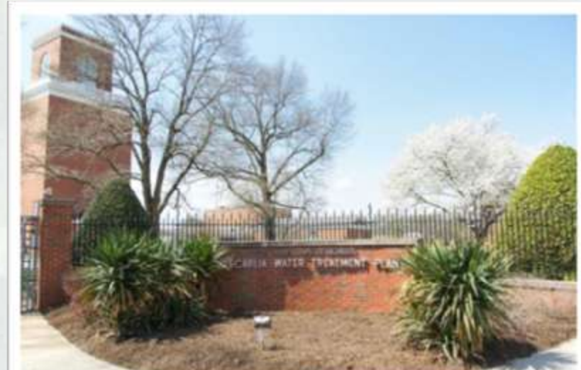
Dalecarlia Water Treatment Plant
