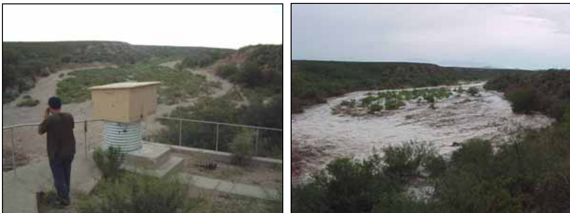
Figure 16. Photographs of Flume 1 at WGEW, dry (left) and with flow (right). (Photographs: USDA/ARS-Southwest Watershed Research Center, Tucson, Arizona)
