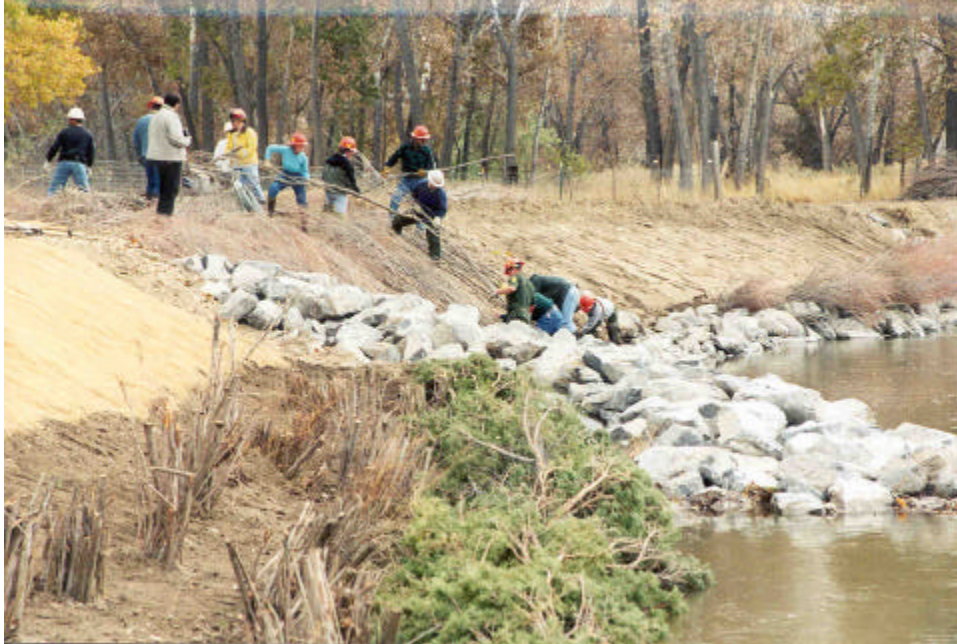
Figure 4. Incorporating irregular alignments, features such as spurs, and other habitat measures into a revetment can significantly improve habitat benefits
