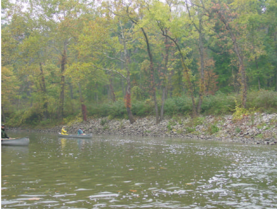
Figure 9. Careful placement of riprap can allow the preservation of mature trees along the banks and avoid impacts associated with their removal
