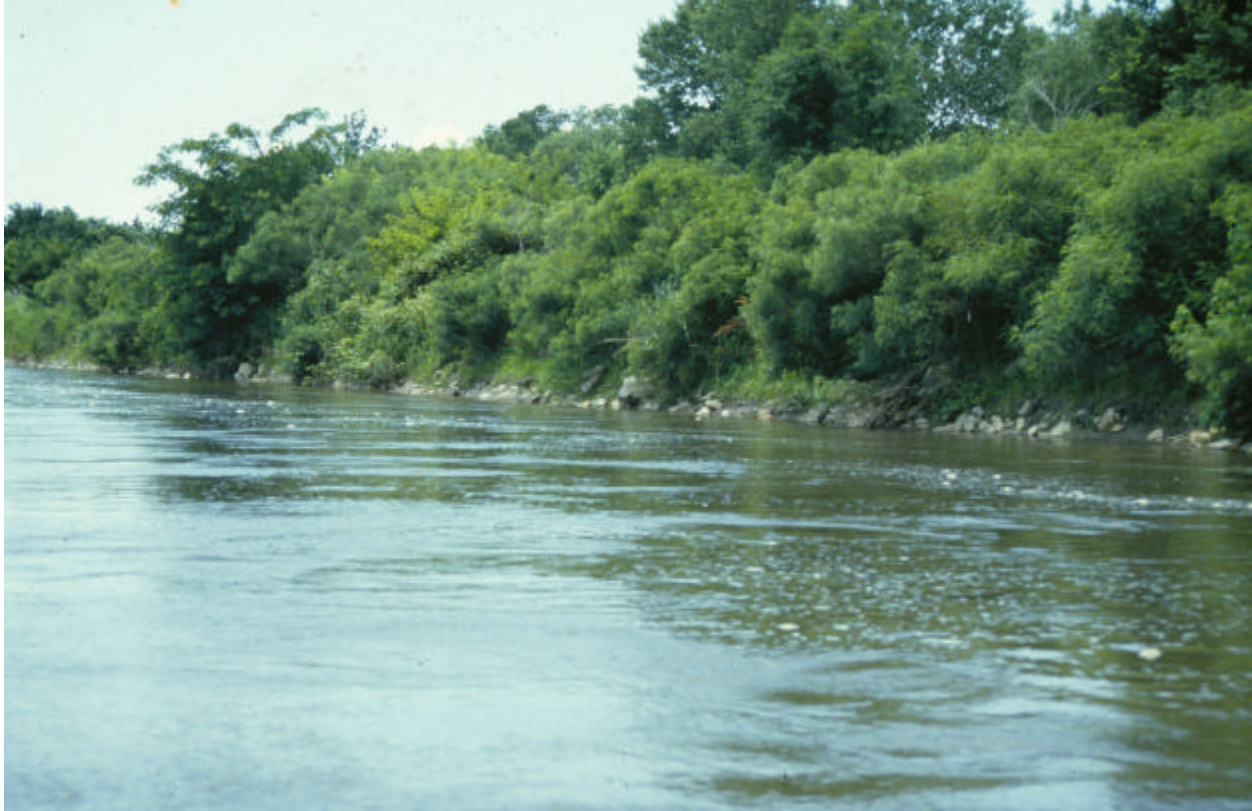
Figure 6. A combination of riprap in the toe section and woody vegetation on the upper banks often affords the best combination of stabilization and environmental benefits
