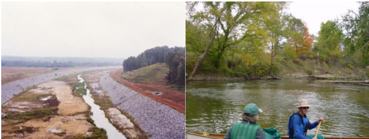
Figure 3. Common problems include setting the riprap elevation higher than needed and not extending the protection far enough downstream
