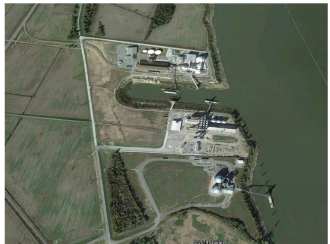
New Madrid County Harbor
