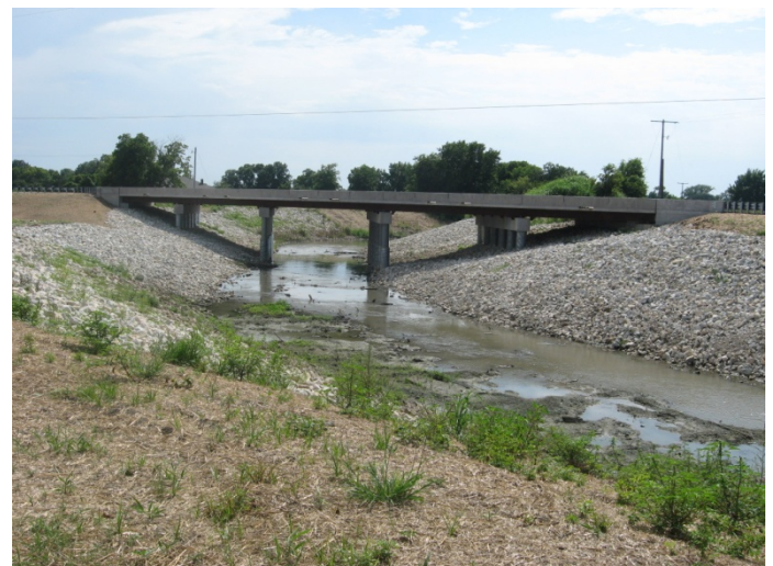
Completed bridge over 15 Mile Bayou on Hwy 147.
