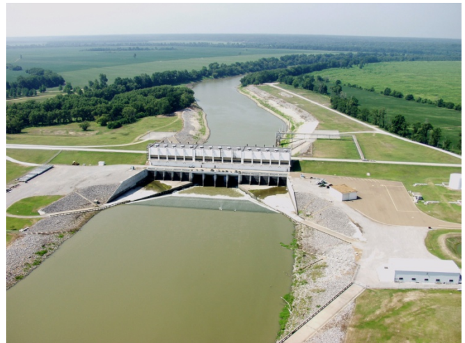
W.G. Huxtable Pumping Plant
