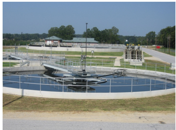
Short Fork Wastewater Treatment Facility
