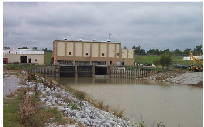
Graham Burke Pumping Station
