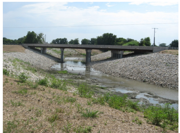
Completed bridge over 15 Mile Bayou on Hwy 147.
