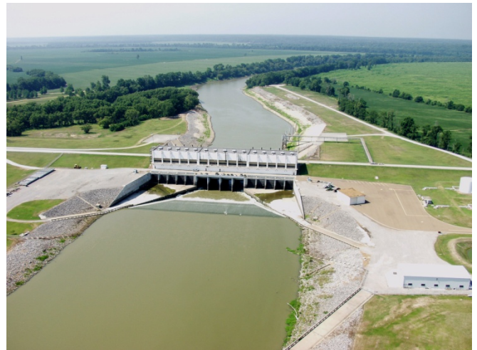
W.G. Huxtable Pumping Plant
