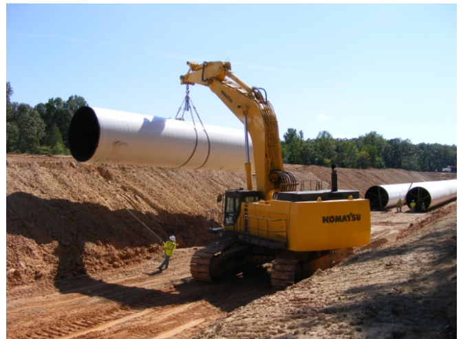
Installation of Grand Prairie Discharge Pipes, Segment 2
