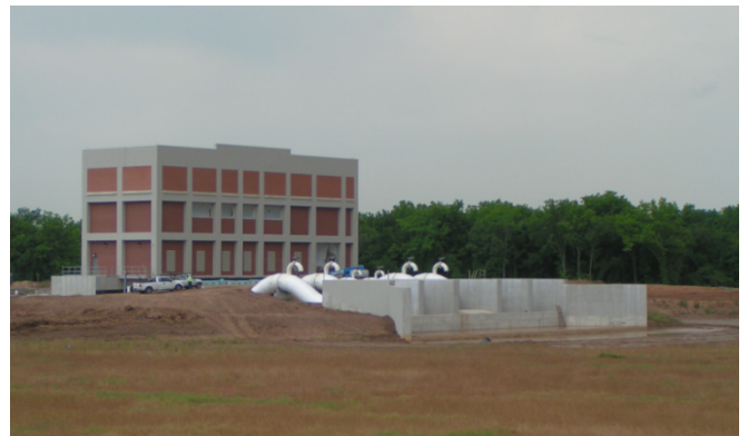
Construction of Pump Station No. 1 (Front/outlet side view)
