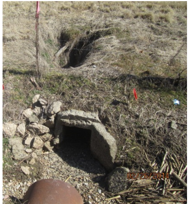
One of several culverts to be replaced along the Farrenburg Levee
