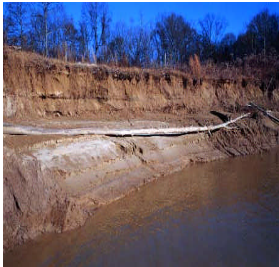
Figure 5. Large woody debris placed by a contractor that has had all limbs removed prior to placement
