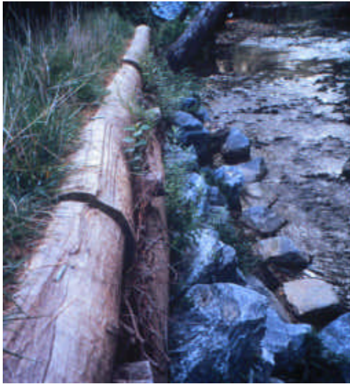
Figure 3. Category 2 LWD structure used to stabilize a stream bank
