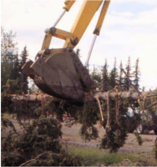
Figure 8. An excavator with a "thumb" used to place LWD
