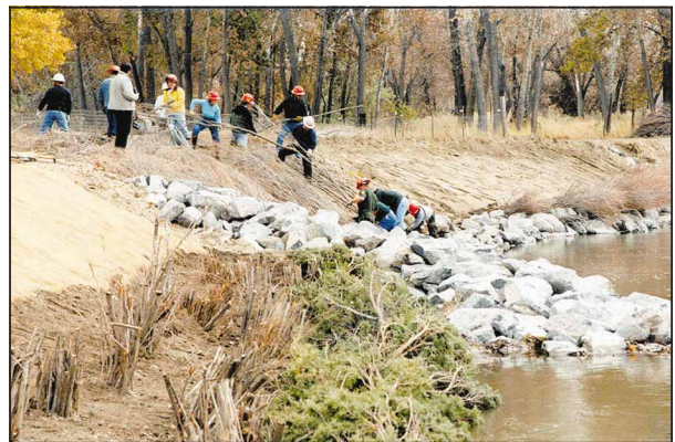
Volunteers installing bioengineering features on a restoration project near Carson, NV
