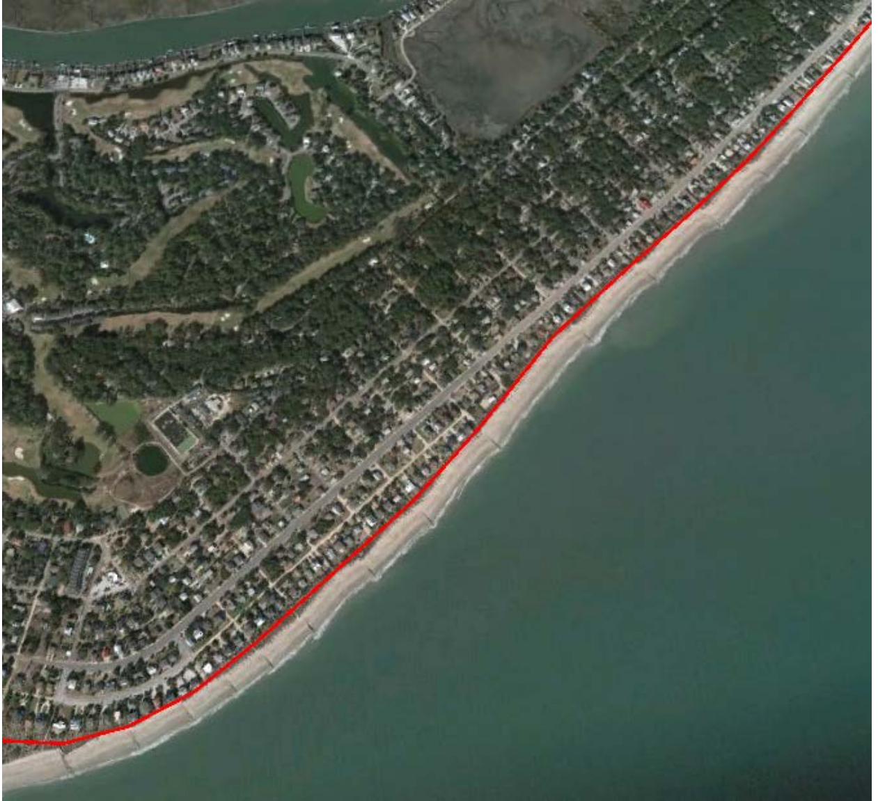
Figure 48: Construction baseline, Reaches P2 and E1 – E6.
