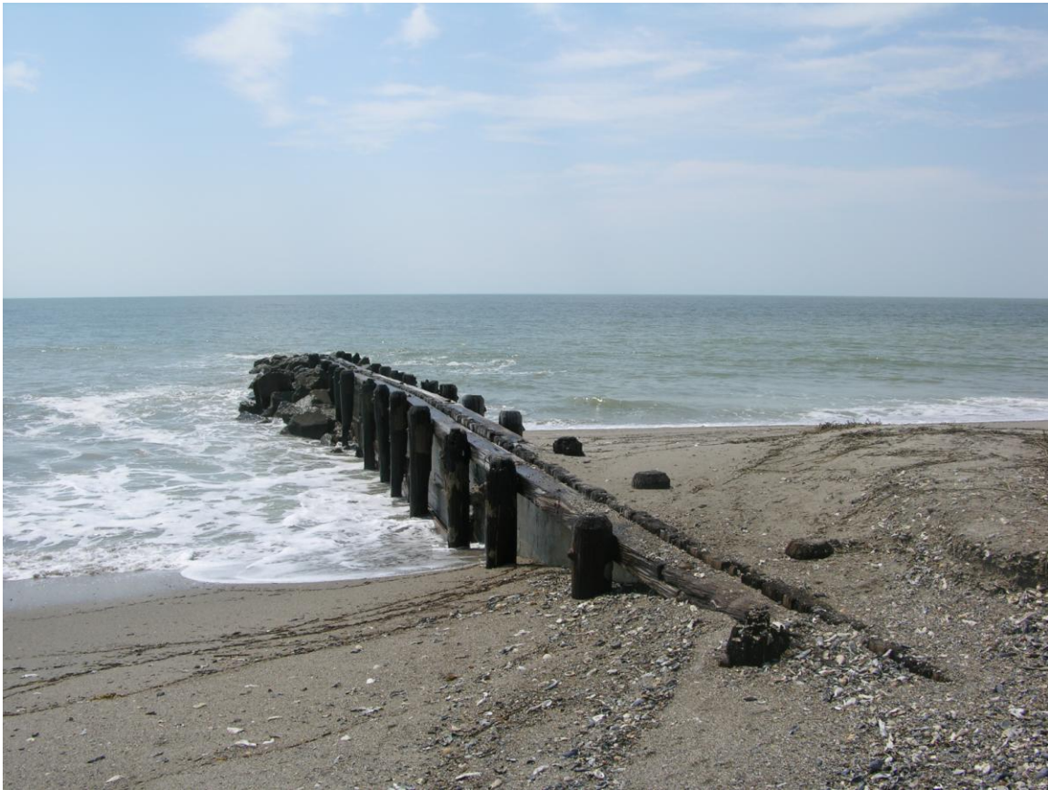
Figure 3.2: Example of one of the 34 groins built on Edisto Island.
