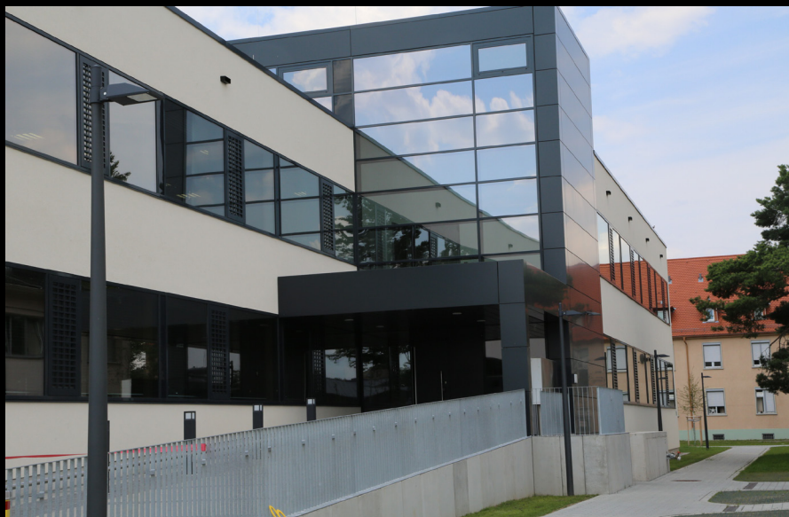
Work ended in April on the Information Processing Center project at Clay Kaserne in Wiesbaden, Germany. Three months ago, the facility was dedicated as Lt. Gen. Robert E. Gray Cyber Center Europe at a ribbon-cutting ceremony.
