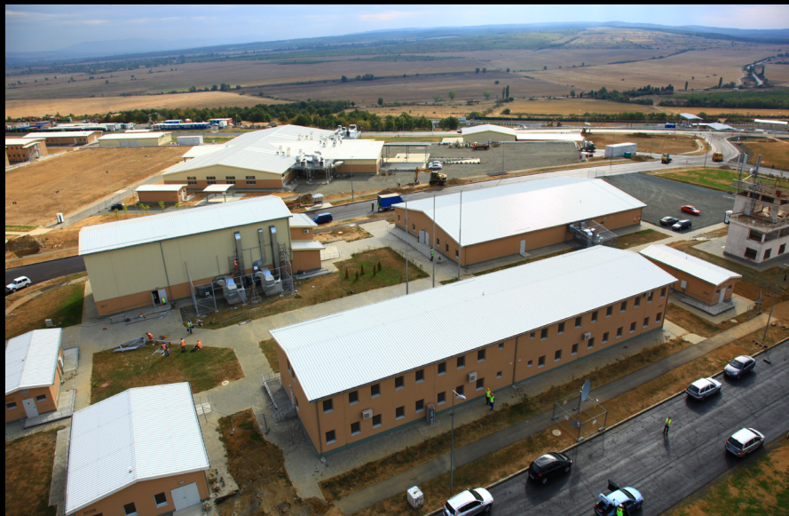
The Bulgaria Project Office continues work at Novo Selo Training Area, a Permanent Forward Operating Site near Mokren, Bulgaria. The office is currently administering contracts to construct a new entrance road for the PFOS and provide a medium-voltage connection point.
