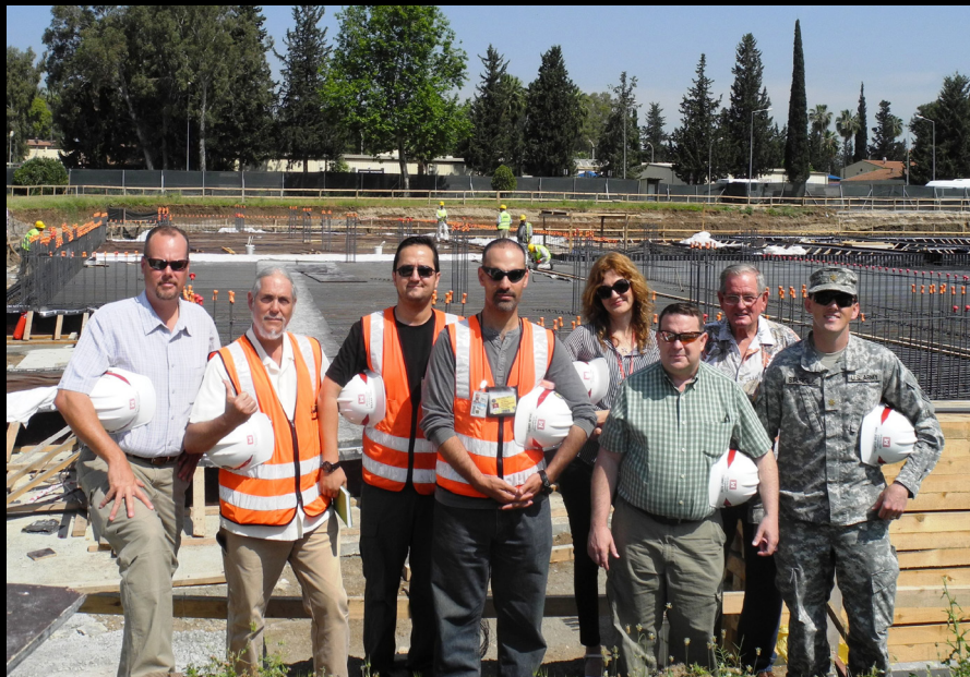
Staff members (from left), pictured recently at the construction site for the Combined Community Center at Incirlik Air Base, are: David Vernon, Francisco Colon, Volkan Tunay, Orkun Dincer, Nilay Yardimci, Tommy Rose, Charles Truesdell and Maj. Josh Sturgill. The new facility is set for completion in 2014.
