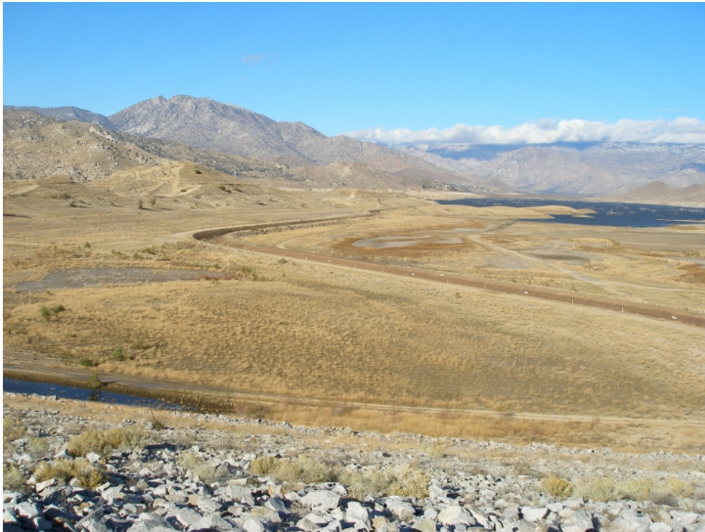
Figure 5. Upstream Portions of the Borel Canal Currently Visible due to Drought-Induced Low Water Conditions in Isabella Lake.
