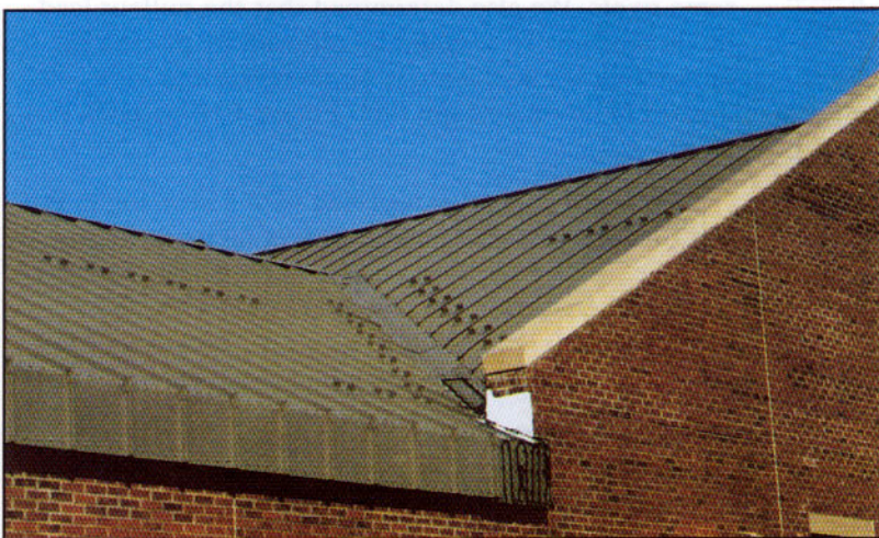
Figure 9: Individual aluminum angle snow guards attached with butyl-based peel-and-stick adhesive.
