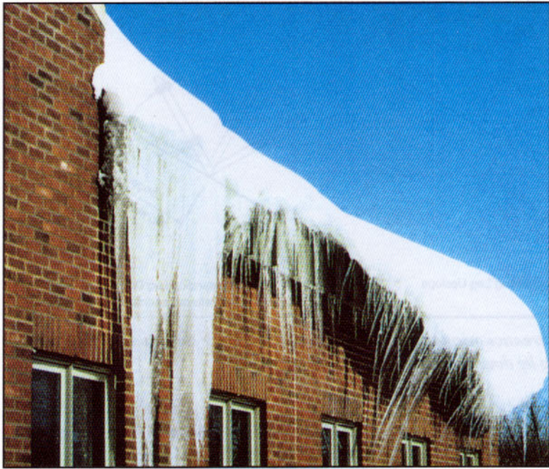
Figure 7: Icicles will form on an overhanging, creeping mass of ice and snow.
