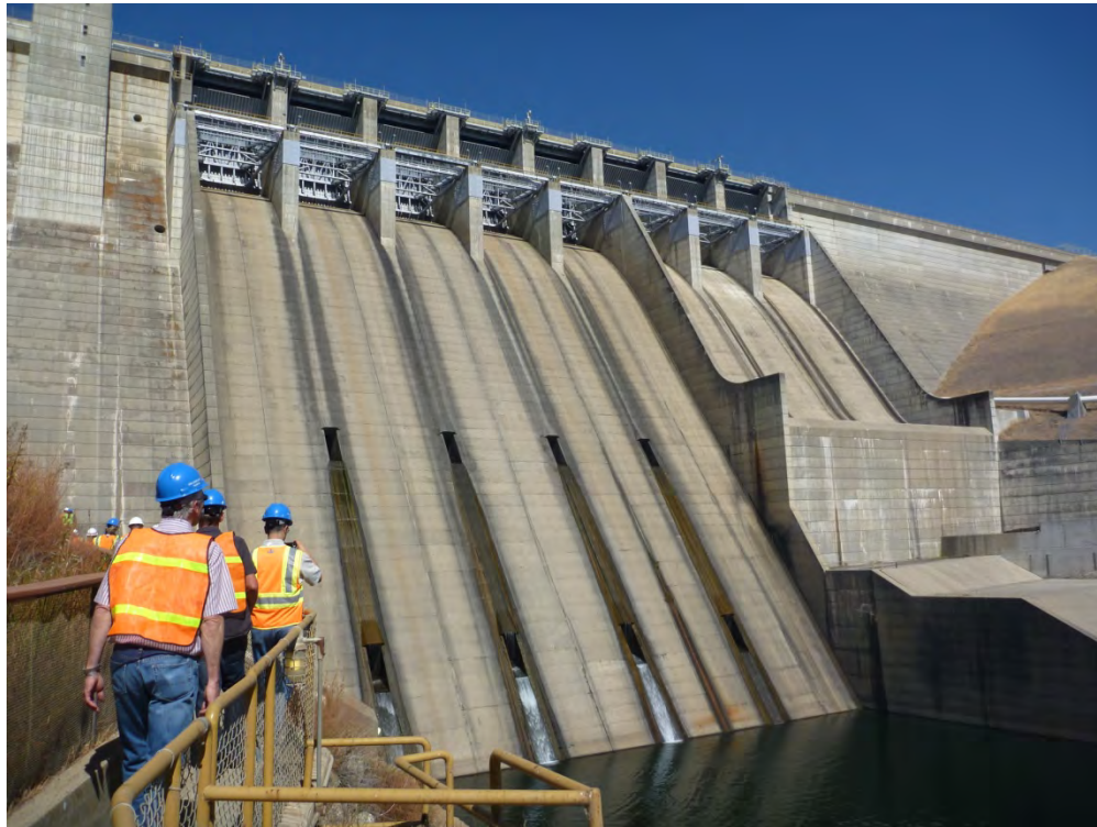
Figure 2. Existing Emergency Spillway Gates (3 on the right)
