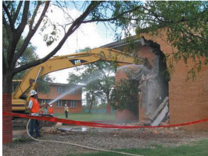
Dorms Demolition Work, FY10 Small Business Award Cannon AFB, Clovis (NM)
