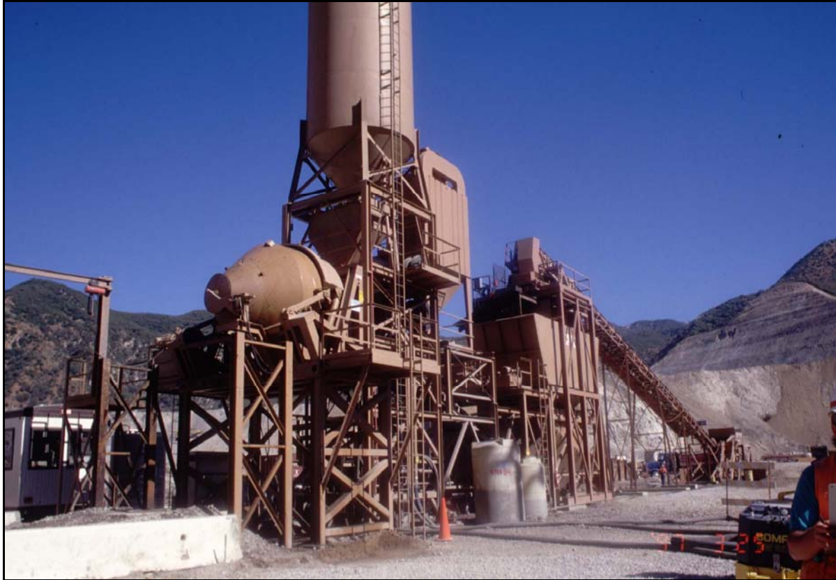
Figure 2-1. Typical Batch Plant.
