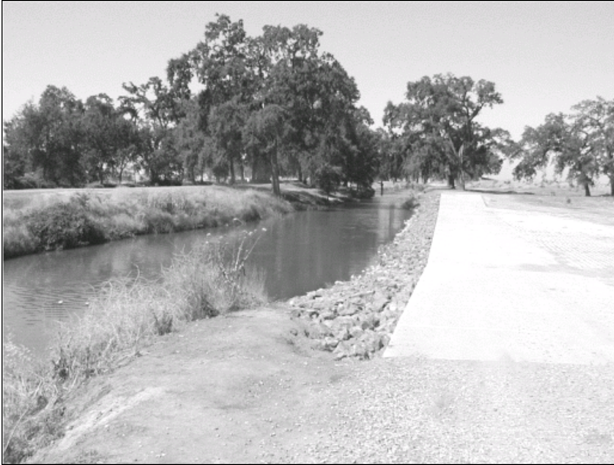
Figure 6. View of Mosher Creek and spillway into SJAFCA Detention Basin #1. This photo is looking west from State Highway 99 across southern edge of existing storm drain detention basin. Noteworthy features are existing riprap bulkhead, concrete pad, and foundation block spillway leading down (north) into the detention basin (not shown).
