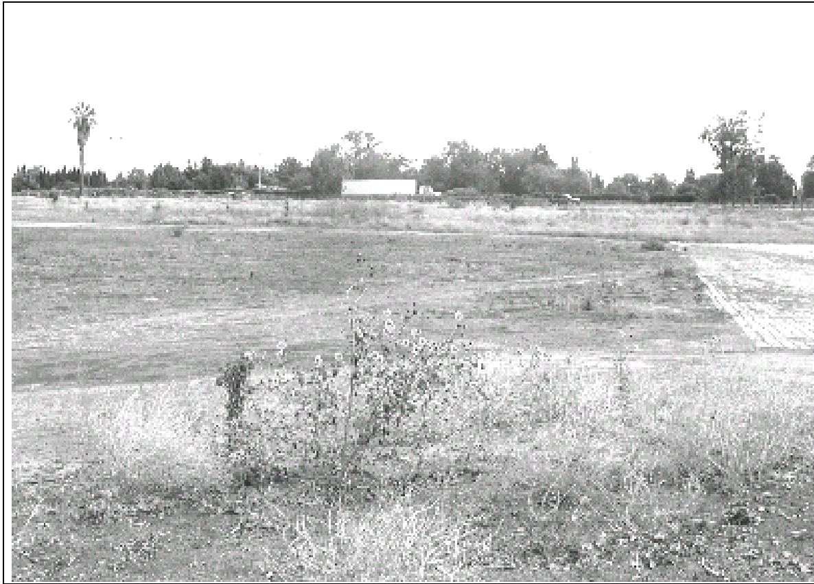
Figure 5. (Cover Photo) View of Demonstration Site #1 looking east across SJAFCA Detention Basin #1 toward State Highway 99. The photos shows the southern edge of basin where proposed 100' by 100' by 2' high berm would be constructed. Noteworthy features are foundation block spillway leading down (north) into the sloping basin and the basin. Levee on eastern perimeter is visible. Vehicles on State Highway 99 are visible in the background.
