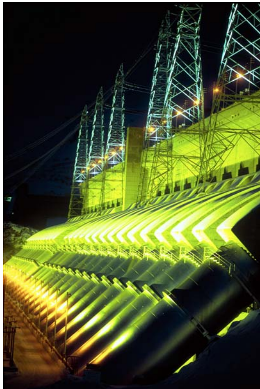
PENSTOCKS LIT DURING THE NIGHT AT CHIEF JOSEPH DAM, WASHINGTON
