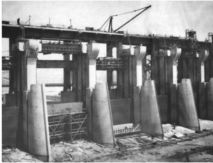
CONSTRUCTION OF FORT PECK DAM, MONTANA
