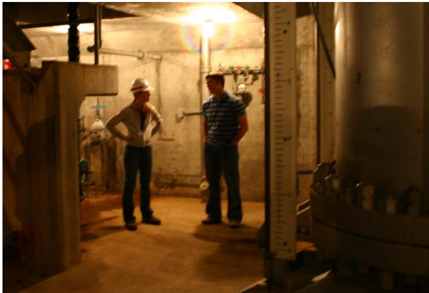
EITs DISCUSS CONDITION IN THE INTAKE TOWER AT COUGAR DAM, OREGON
