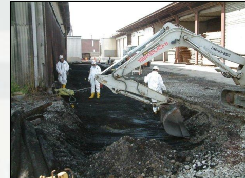
Remediation at FUSRAP St. Louis Downtown Sites
