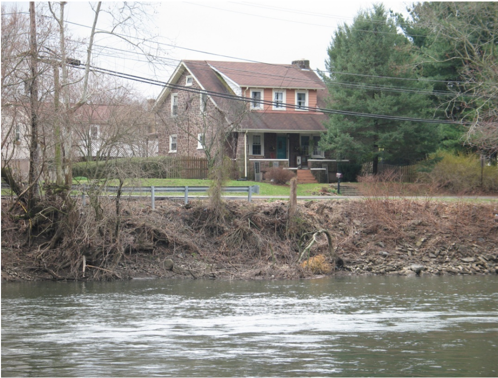
Figure 3. View of project area from the opposite streambank (Photo 2008).
