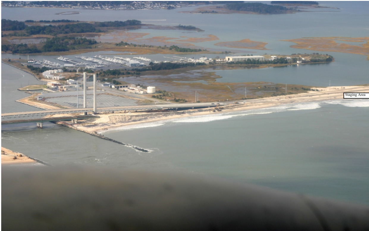
Photo 5: Indian River Inlet project area showing beach staging area
