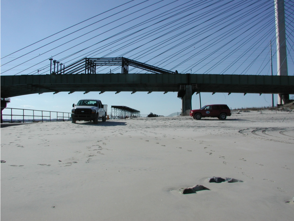
Photo 3: North Shore Beach Existing Conditions (under bridge) (February 12, 2013).
