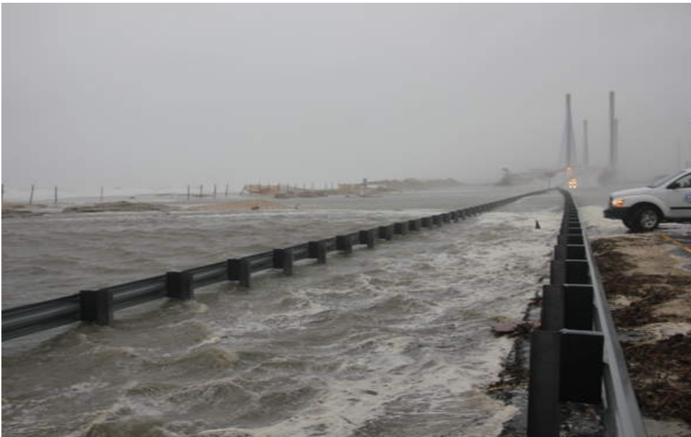
Photo 2: State Route 1 and Indian River Bridge during a recent storm (water pooling) (March 6, 2013).
