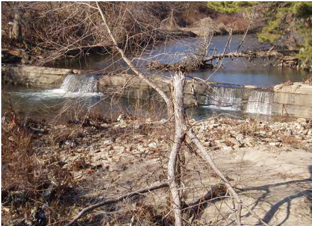
Figure 4. Woodland Dam shown from the Woodland Avenue Bridge approximately 200 feet downstream of the dam.
