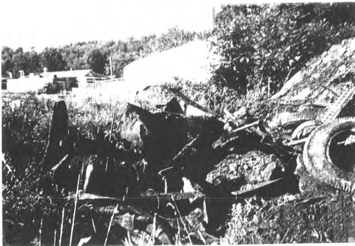
PHOTOGRAPH 25 - 9/16/97 Metal rails, basins, other debri from L-M area excavation
