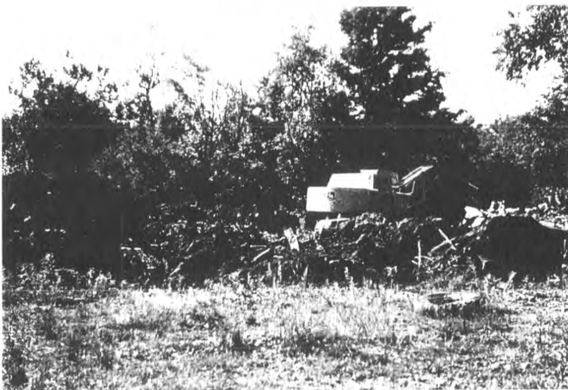
PHOTOGRAPH 45 - 9/16/97 Soil & debris piles from long excavation East of Willowemoc Creek
