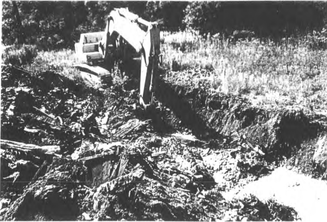
PHOTOGRAPH 37 - 9/16/97 Excavation from P-0 to O-25-: plastic, trash & wood
