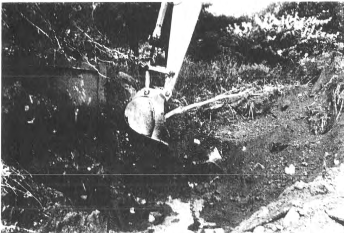
PHOTOGRAPH 40 - 9/16/97 Excavation from H-25 to I-0
