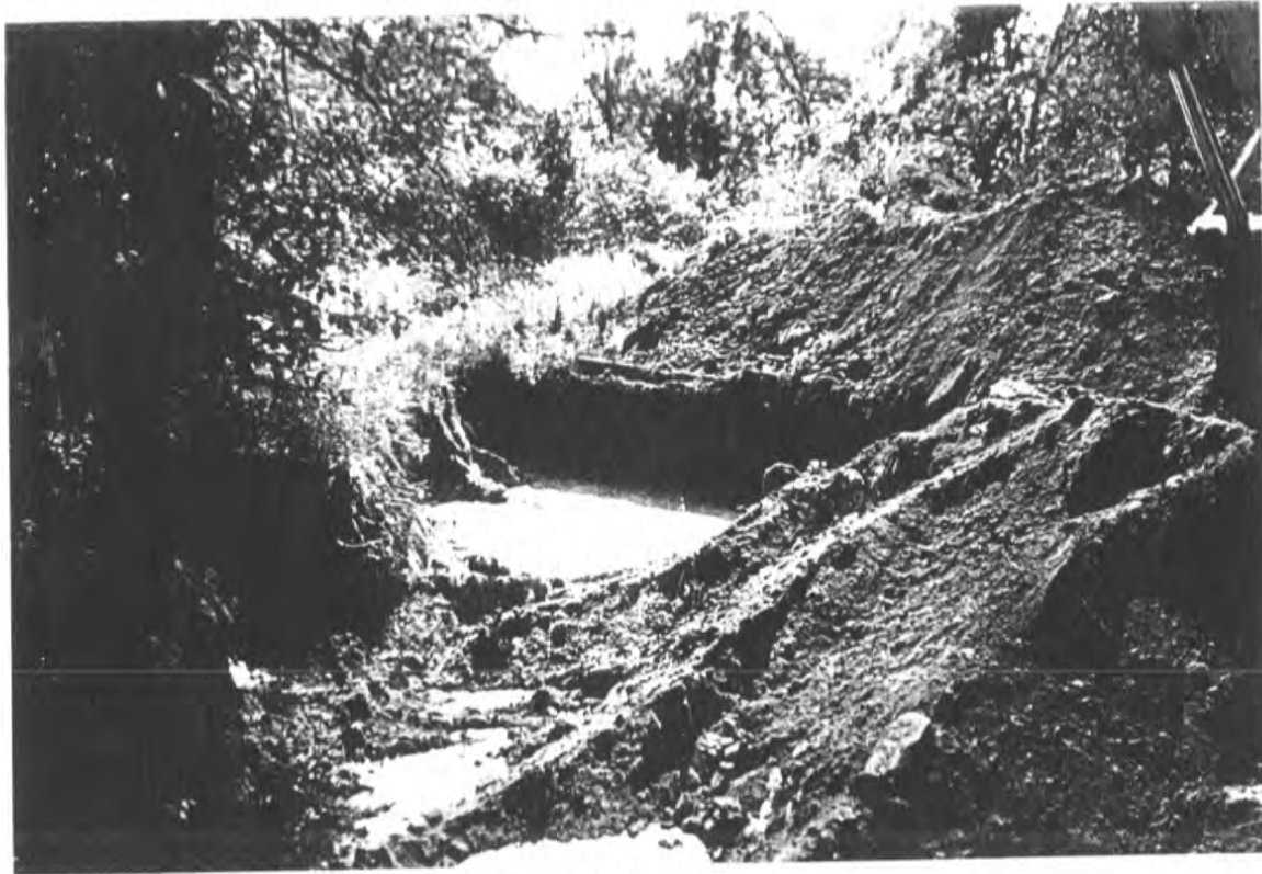
PHOTOGRAPH 1 - 9/15/97 Excavation behind building foundation (O-100 & P-150)
