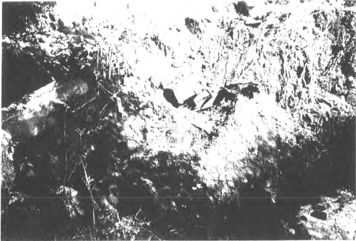
PHOTOGRAPH 41 - 9/16/97 Metal parts & cement along sidewall at I-0
