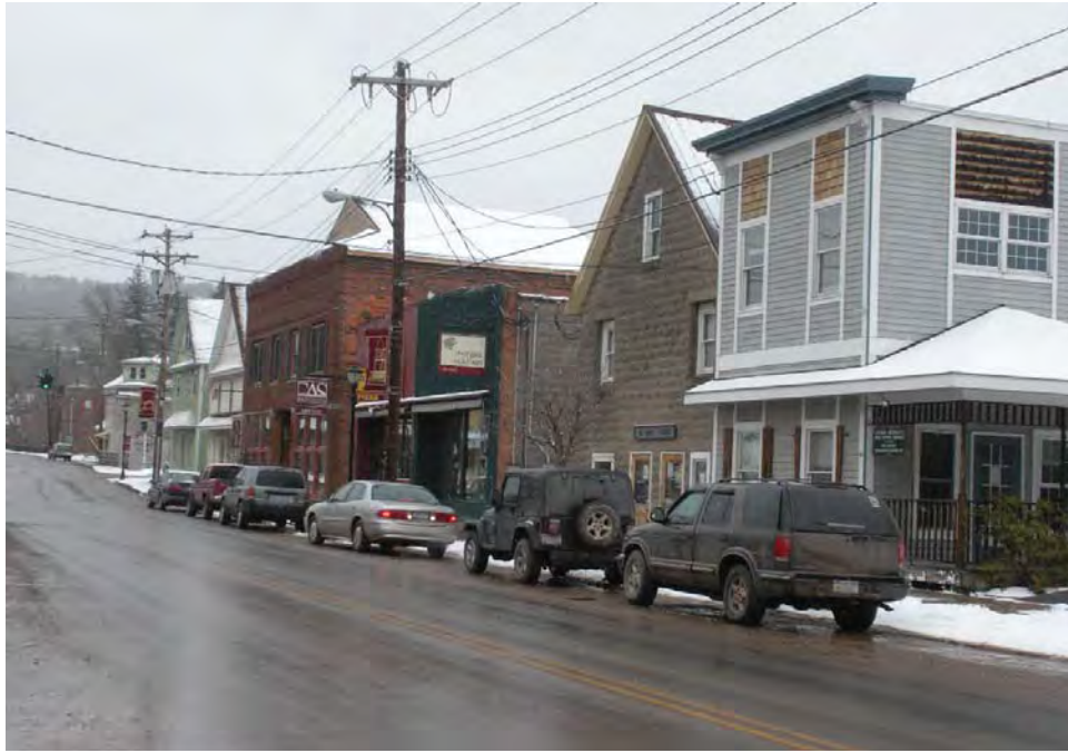
Photograph 15: View facing southwest showing buildings along the west side of Main Street (A016 to A023). The bridge over Little Beaver Kill is located at the left side of the photograph, near the traffic signal, and represents the south end of Area 6 and the center of Area 7 (February 2010).
