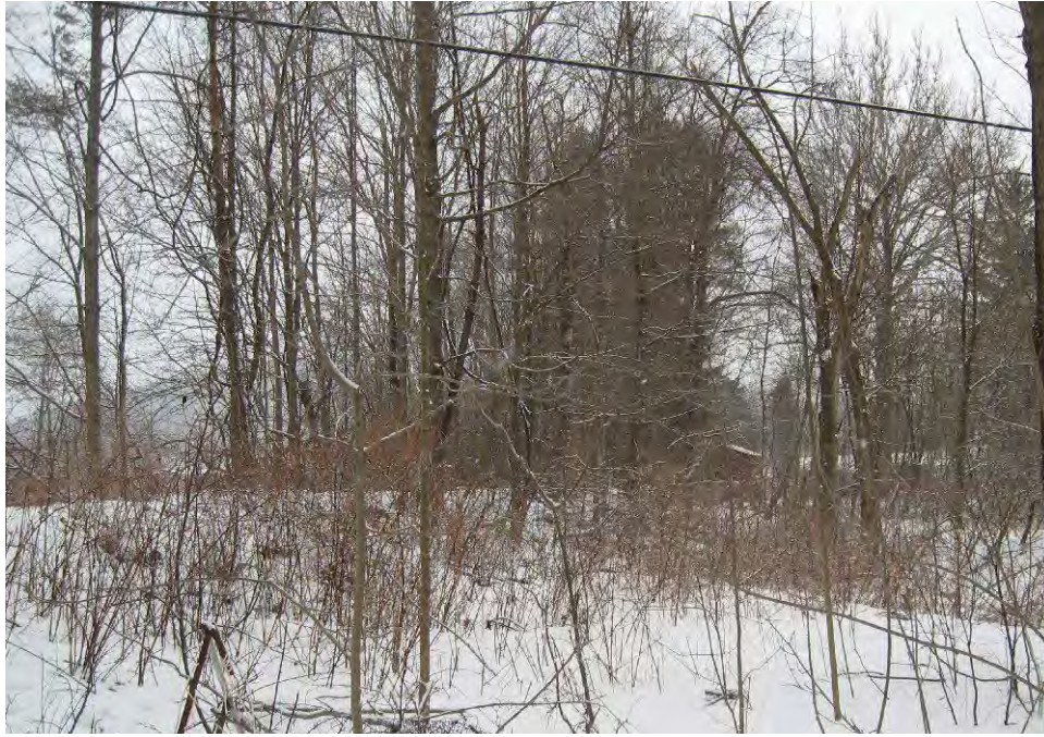
Photograph 13: Earthen berm/levee along the southwest bank of Willowemoc Creek in Area 5. Facing east (February 2010).
