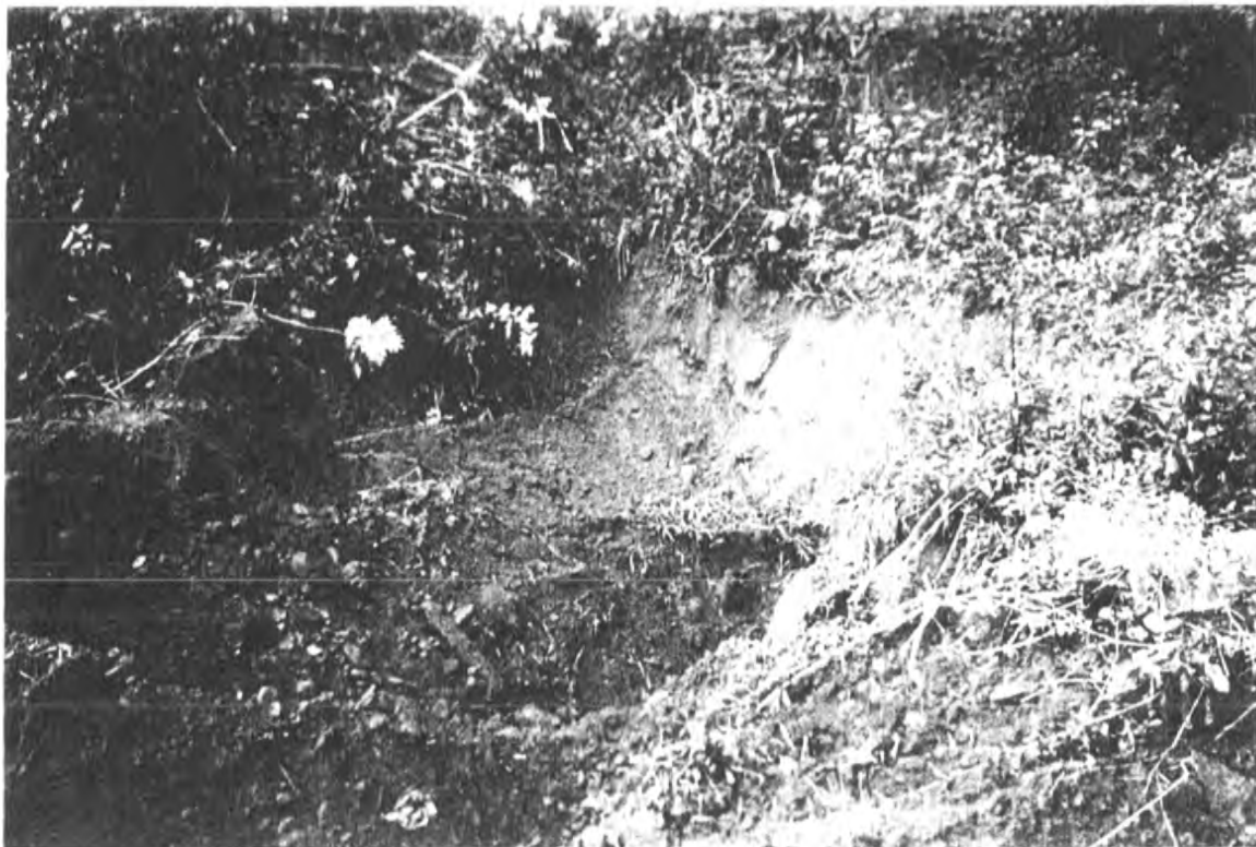
PHOTOGRAPH 20 - 9/16/97 Excavation at L-50-, North of tank enclosure
