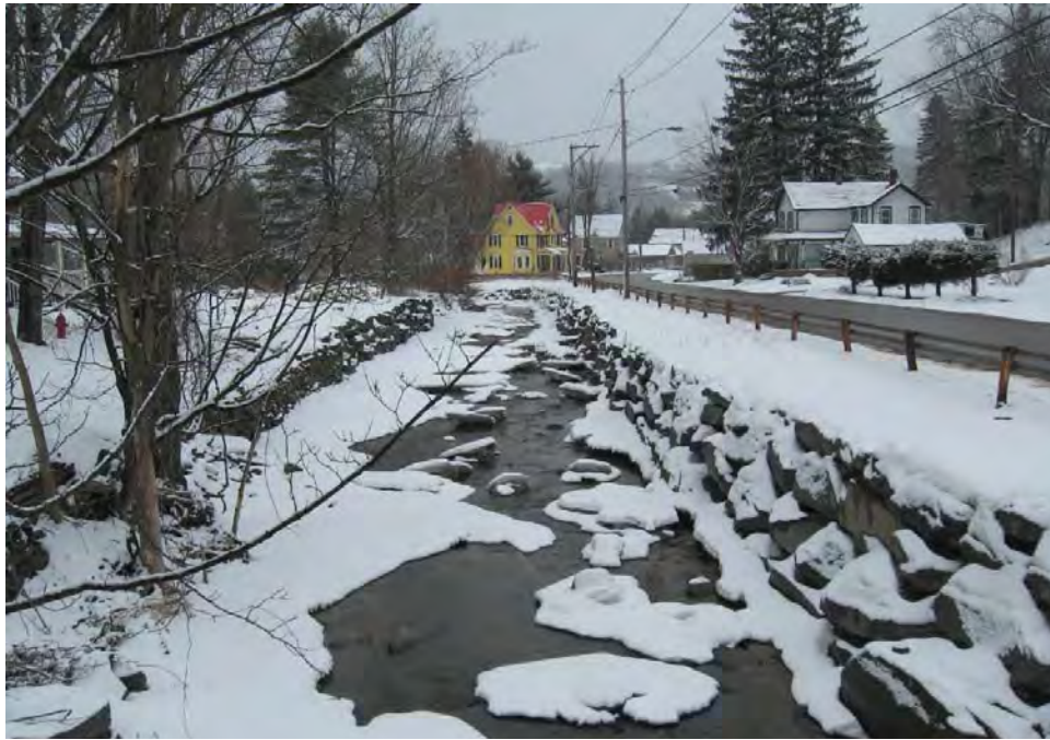
Photograph 33: View of channelized bed of Cattail Brook in Area 10, which runs along the west side of Main Street through most of the project area. Facing northeast toward Church Street and the house at 108 Main Street (A057) (February 2010).
