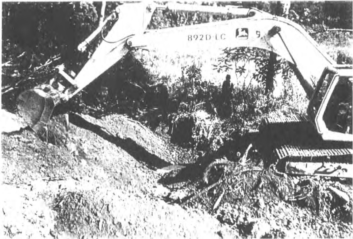
PHOTOGRAPH 29 - 9/16/97 Excavating at L-M area
