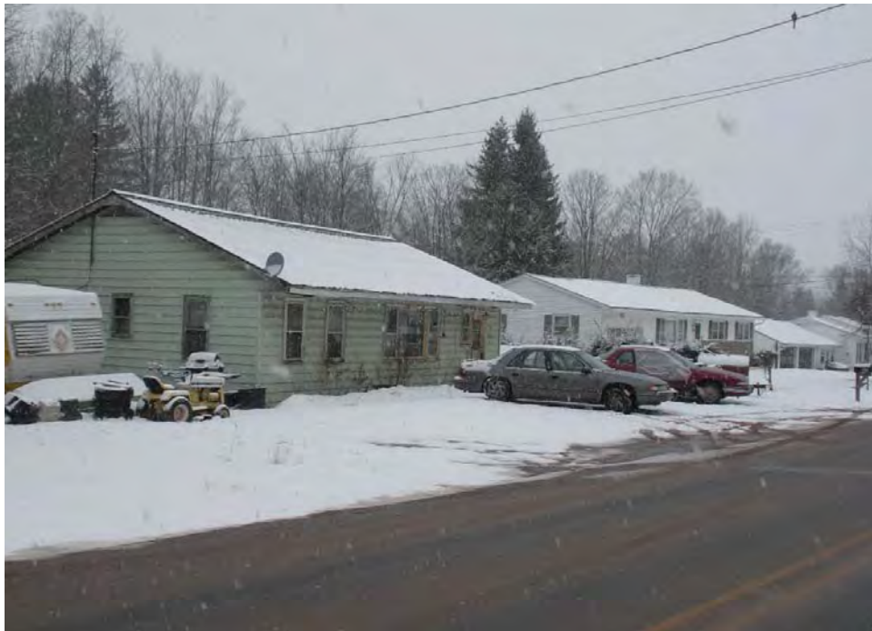
Photograph 36: View of typical mid-twentieth-century buildings at the south end of Area 10 (A068). Facing north along Main Street near the crossing of Cattail Brook (February 2010).
