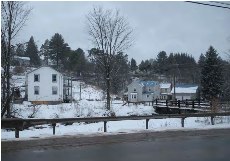
Photograph 34: View of typical early-twentieth-century buildings within Area 10 (A058 to A061). Facing northwest toward Willoughby Street across Main Street and Cattail Brook (February 2010).
