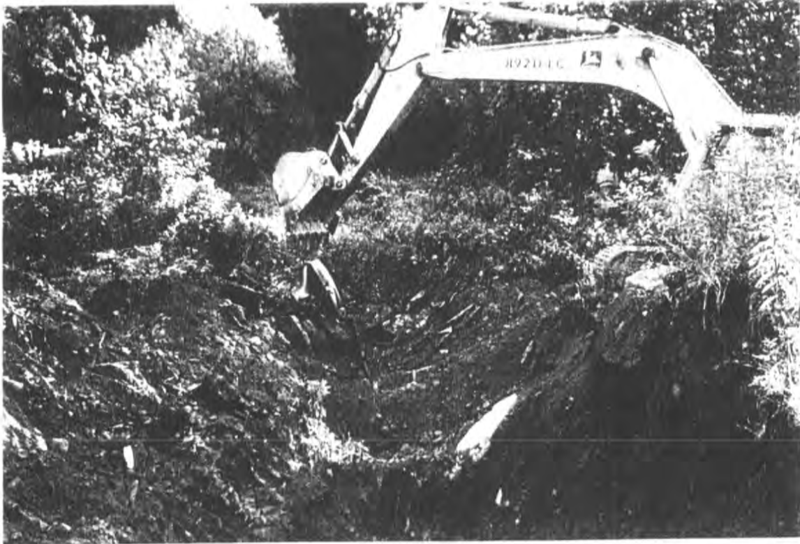
PHOTOGRAPH 46 - 9/17/97 Excavation into bank East of K-130, metal parts
