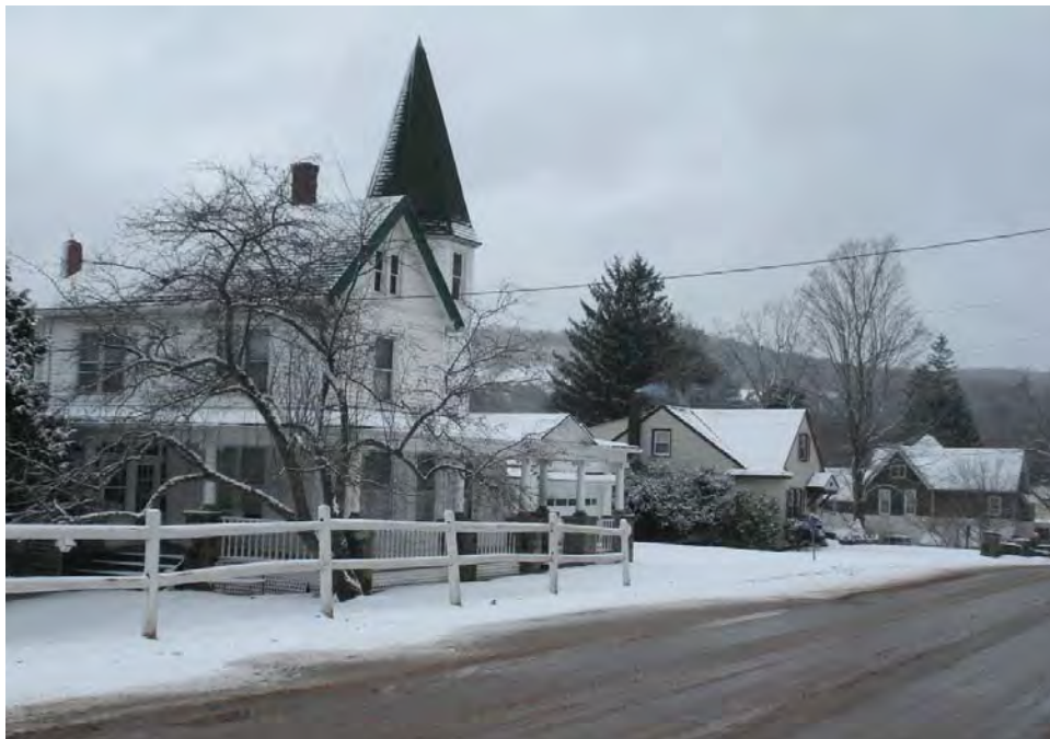
Photograph 26: View of typical buildings along the south side of Pearl Street within Area 8 (A045 to A048). The dwelling at the left, 48 Pearl Street (A048), has been previously documented and is a rare example of Queen Anne architecture within the project area. Facing west (February 2010).
