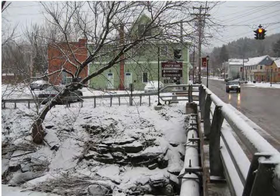
Photograph 18: View of the north quadrant of Area 7 and the parking lot in Area 6. The parking lot is sitting directly above exposed bedrock along the eastern shore of the Little Beaver Kill. Facing northeast (February 2010).
