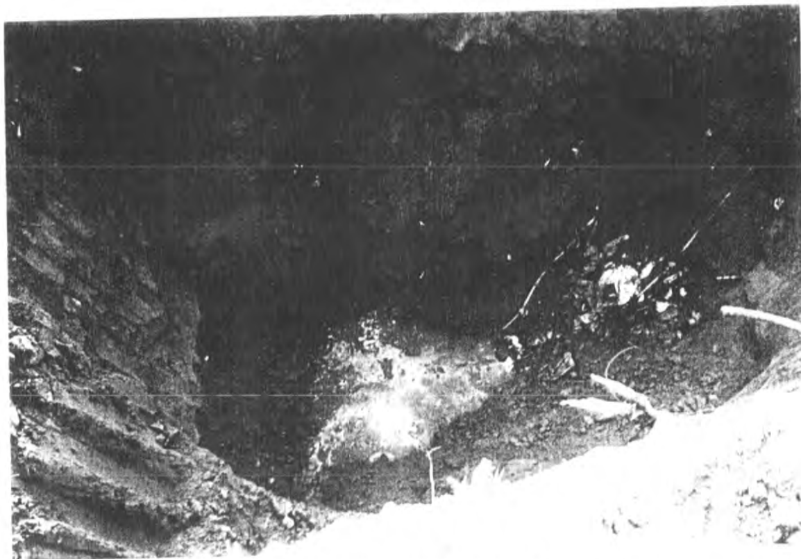
PHOTOGRAPH 2 - 9/15/97 Excavation behind building foundation, note darker soils at water table
