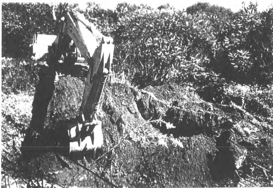
PHOTOGRAPH 13 - 9/15/97 Extend Excavation East toward wetland
