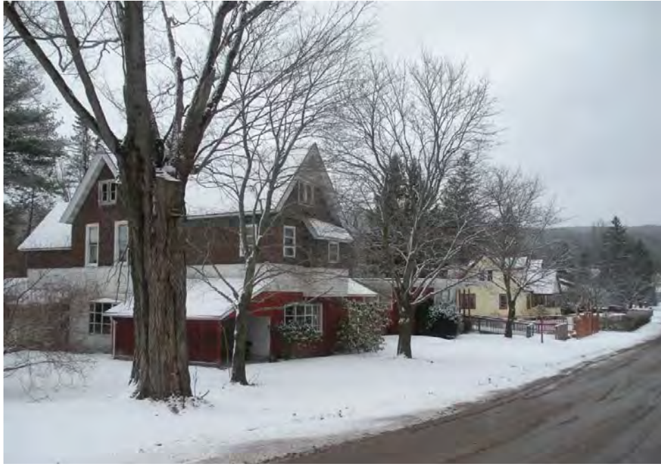
Photograph 25: View of typical buildings along the south side of Pearl Street within Area 8 (A044 and A045). Facing west (February 2010).
