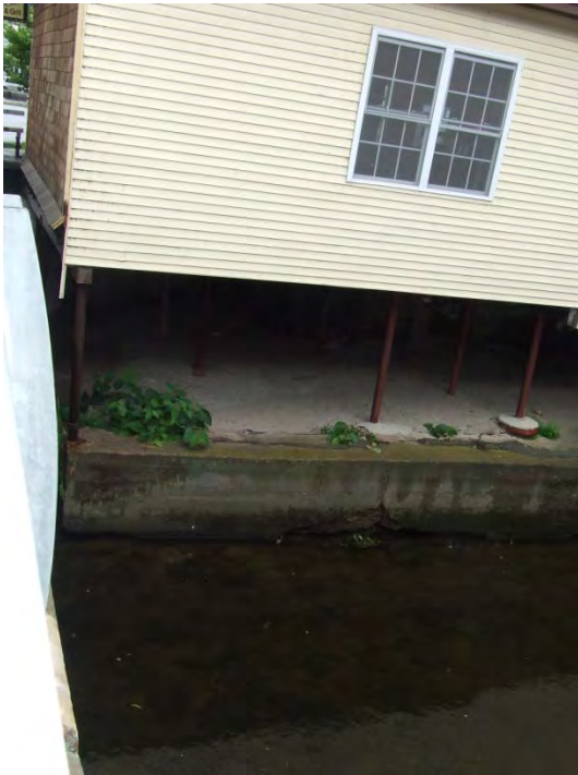
Figure 11.1 - Building on ROB Upstream of Main Street Bridge
