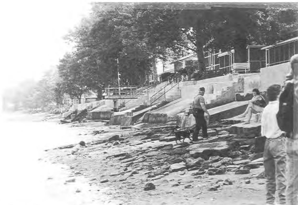
Photo #17: Southern 1/3 of beach. Note the step and wall extensions to the vertical concrete wall undertaken by local residents as sand was lost through the years.
