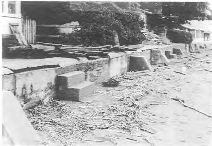
Photo #15: Northern 1/3 of beach. Note the steps adjacent to the concrete wall and the vertical erosion of the beach.
