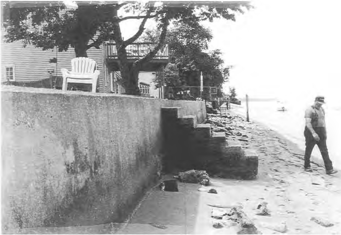
Photo #15: Northern 1/3 of beach. Note the steps adjacent to the concrete wall and the vertical erosion of the beach.
