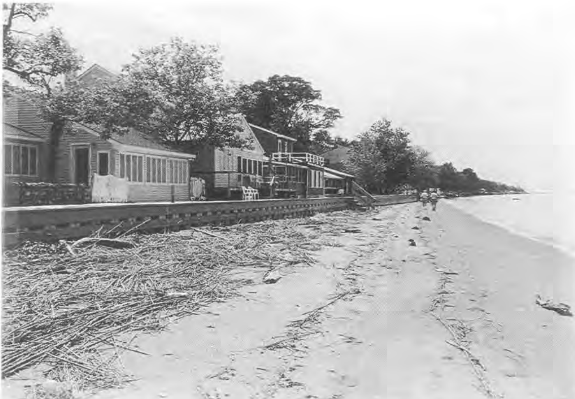
Photo #8: Natural beach area in November 1996 protected by Shore Guard vinyl sheetpile bulkhead (middle 1/3 of beach).
