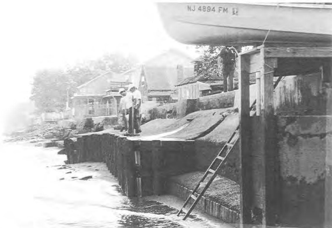
Photo #9: Southern 1/3 of beach. Note the staged construction of the protective structures undertaken by individual homeowners. Note the vertical concrete wall fronting the properties, followed by a sloped concrete wall, followed by a timber bulkhead.
