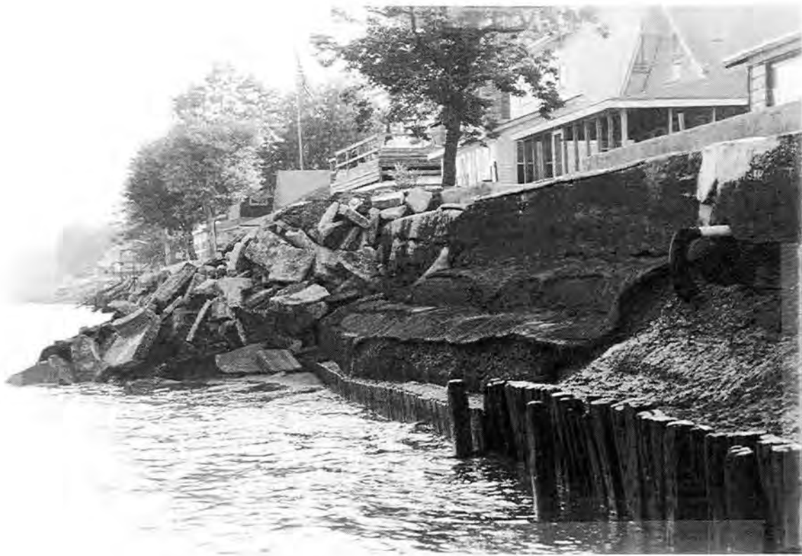
Photo #1: Sloped concrete wall fronted by timber bulkhead (southern 1/3 of beach).
