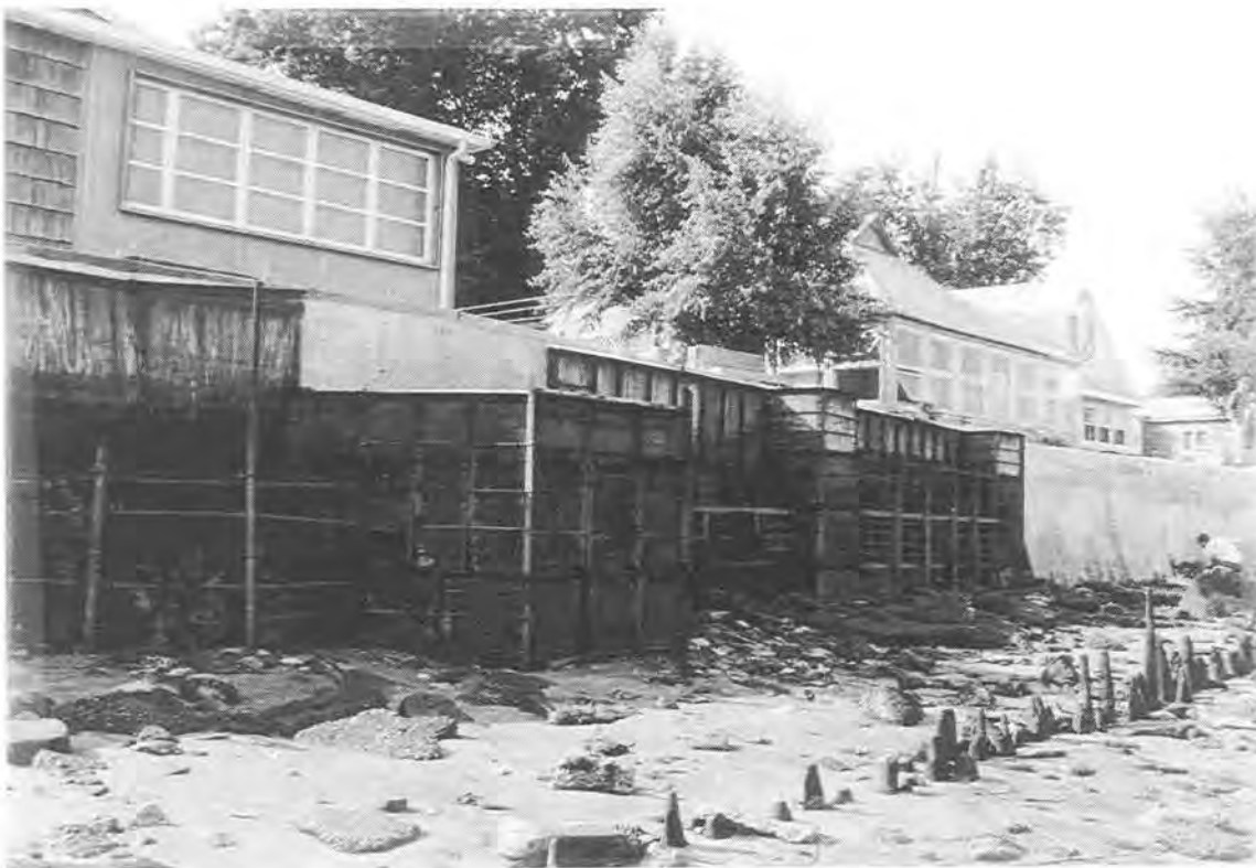
Photo #14: Southern 1/3 of beach. Note the remains of a crude bulkhead in the foreground.
