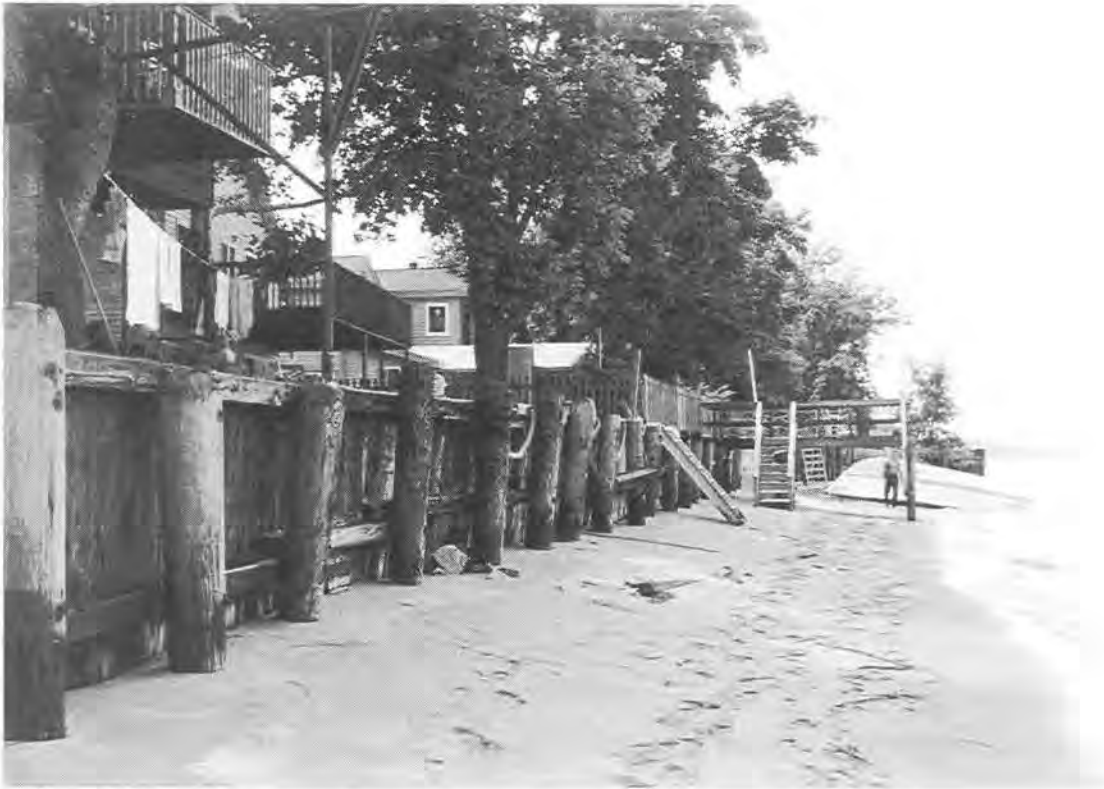
Photo #7: Timber bulkhead (middle 1/3 of beach).
