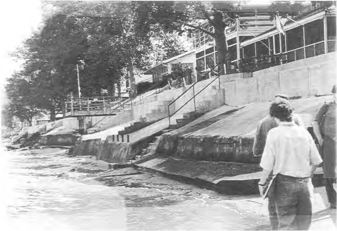
Photo #5: Sloped concrete walls (middle 1/3 of beach).
