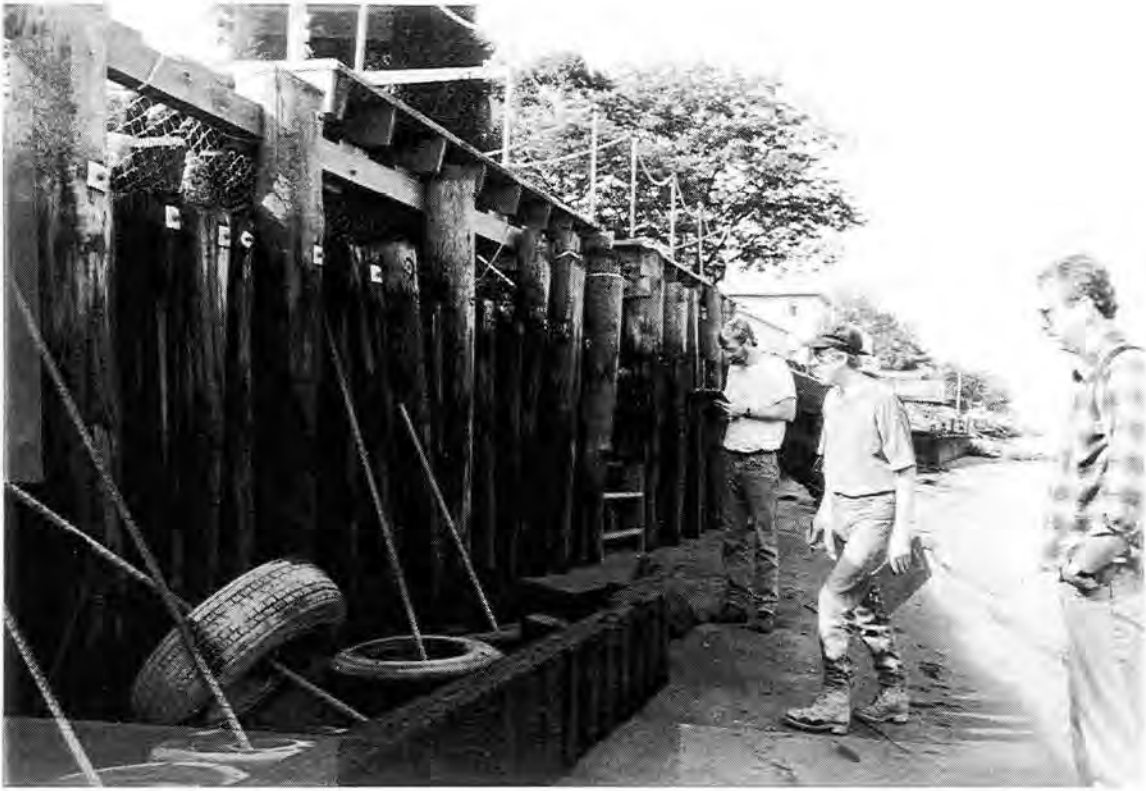
Photo #3: Timber bulkhead (middle 1/3 of beach).
