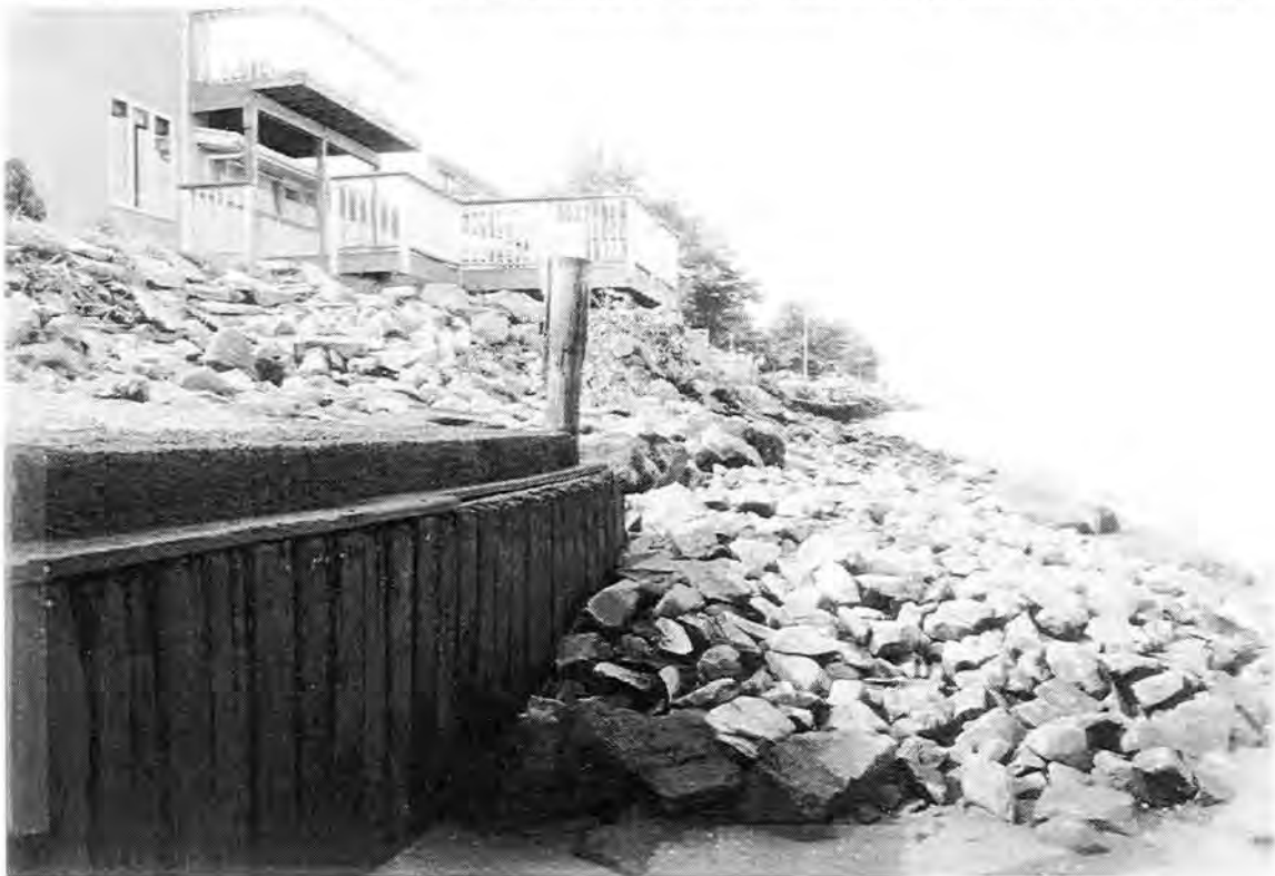
Photo #2: Stone revetment (southern 1/3 of beach).
