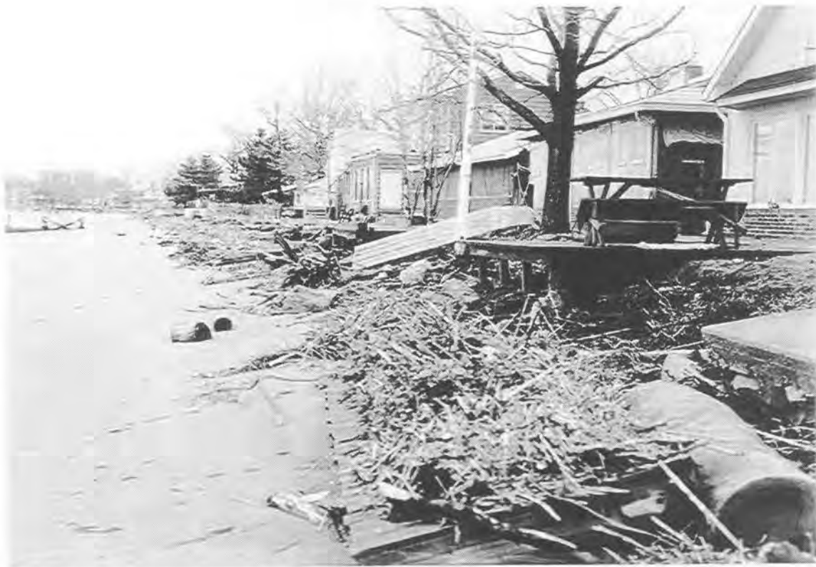
Photo #19: Middle 1/3 of beach. Unprotected beach area following March 1996 storm. Note the debris and deck damage and the undermining of the structures. Following this storm, local residents bulkheaded the area (refer to Figure 12, photo #8).
