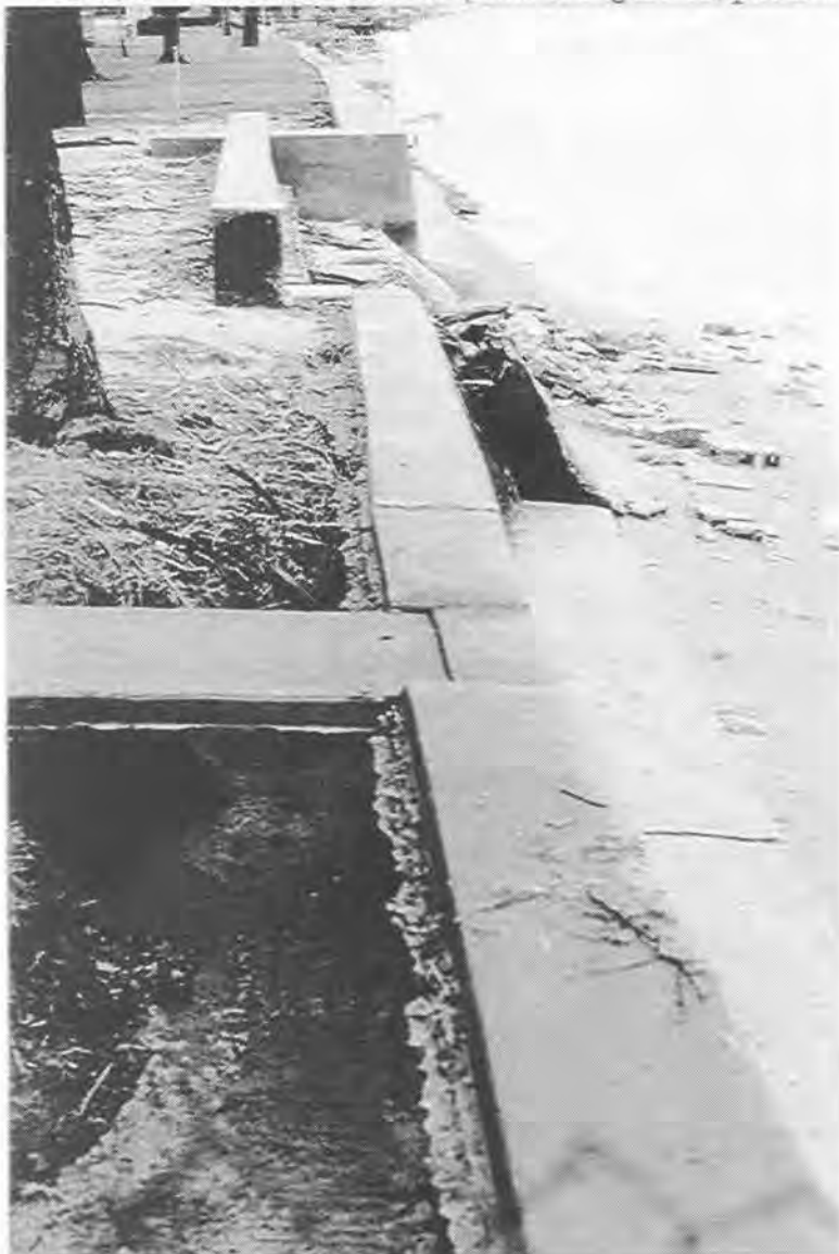
Photo #19: Middle 1/3 of beach. Unprotected beach area following March 1996 storm. Note the debris and deck damage and the undermining of the structures. Following this storm, local residents bulkheaded the area (refer to Figure 12, photo #8).
