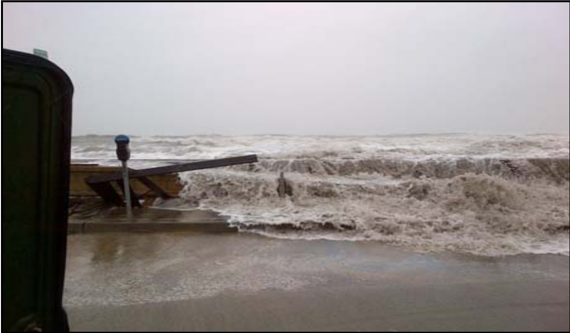
Figure 48 Bulkhead Overtopping During Hurricane Sandy North Wildwood
