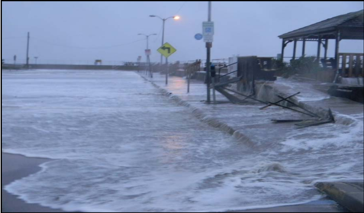
Figure 48 Bulkhead Overtopping During Hurricane Sandy North Wildwood
