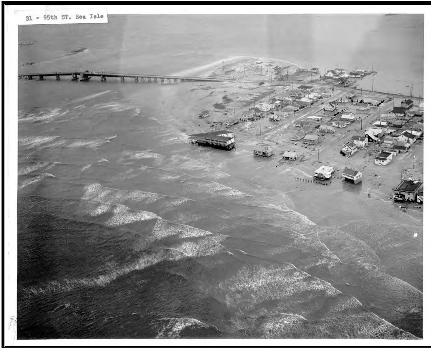
Photo 3-24 Sea Isle City (95 th Street), NJ. Storm of 1962.
