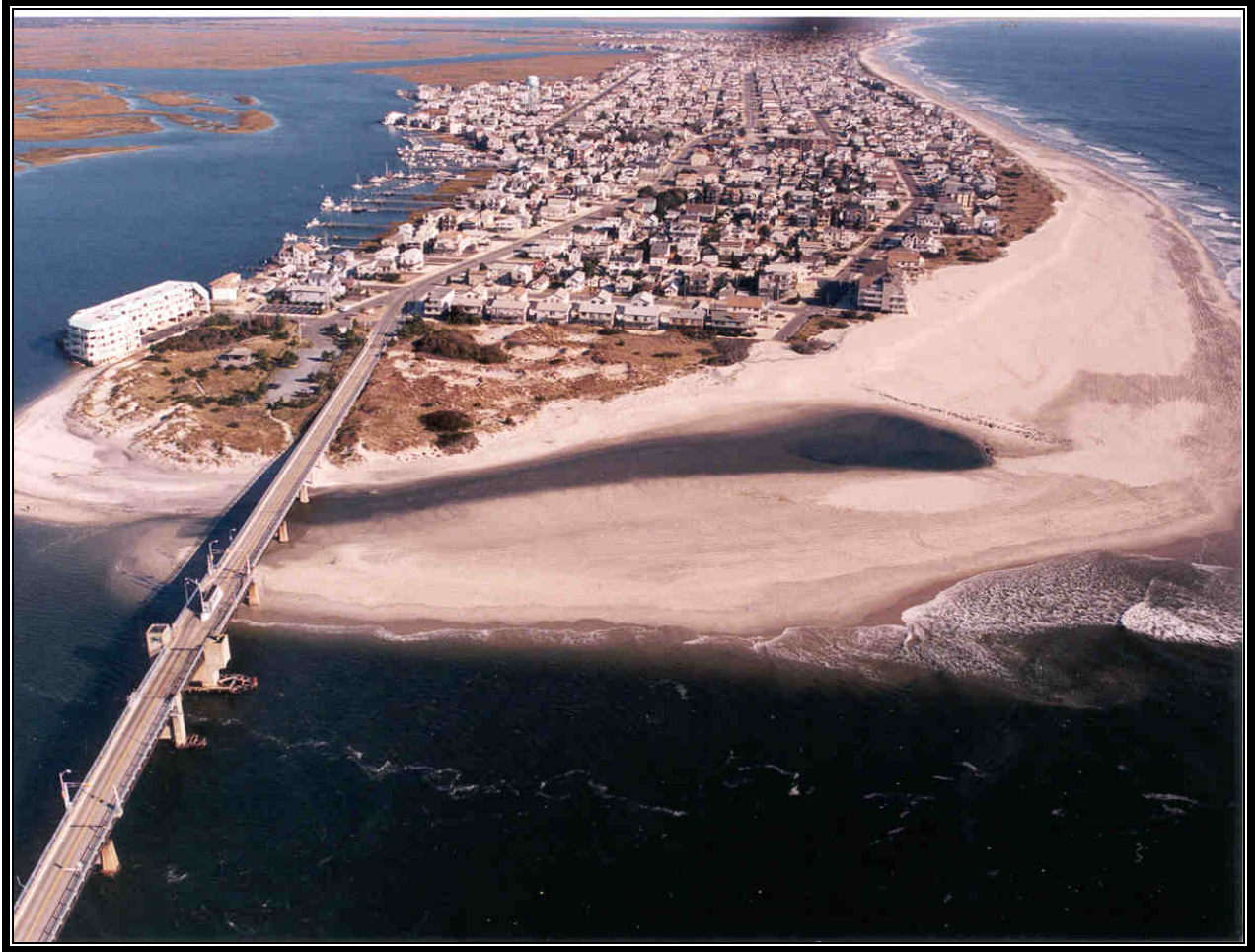
Photo 1-11 Townsend's Inlet area of Sea Isle City, NJ, 10/25/99. Following construction of terminal groin and beachfill placement by locals.
