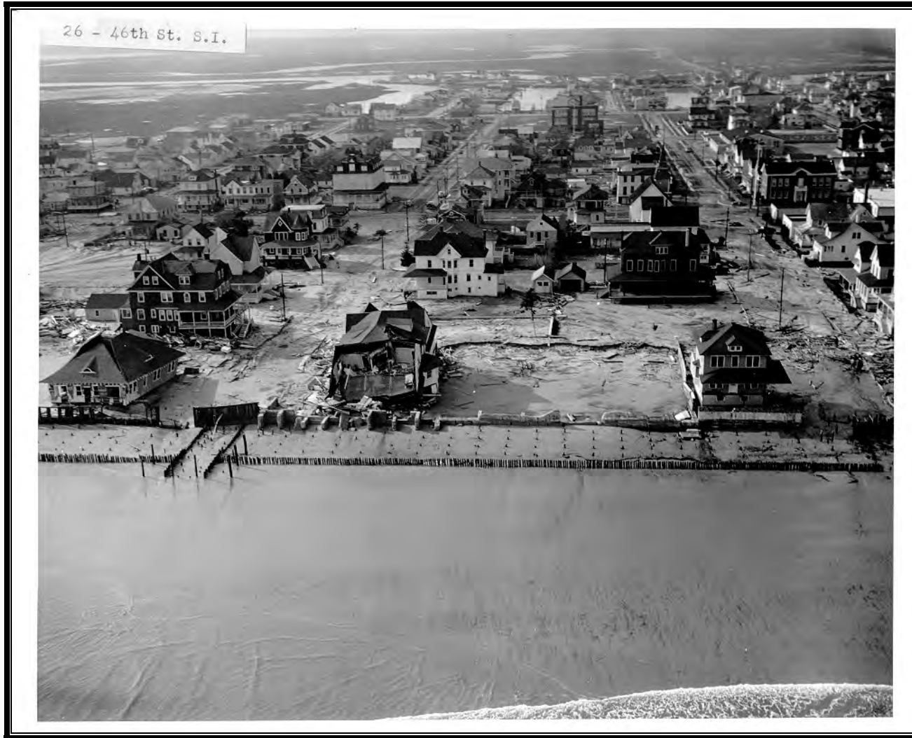
Photo 3-22 Sea Isle City (46 th Street), NJ. Storm of 1962.
