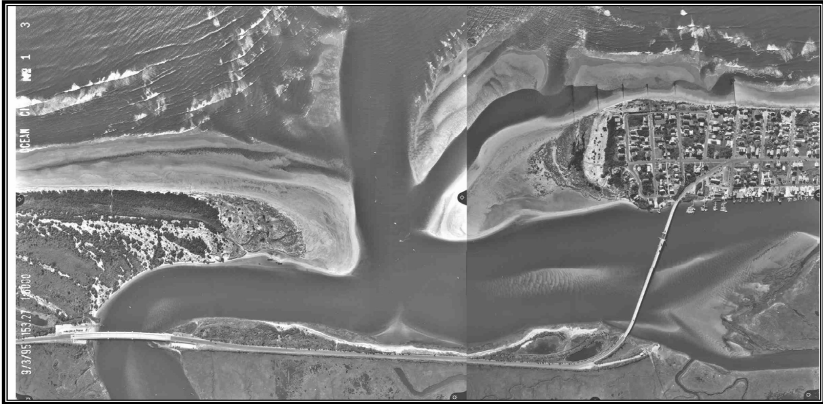
Photo 2-6 Aerial Photography of Corson Inlet (September 1995)
