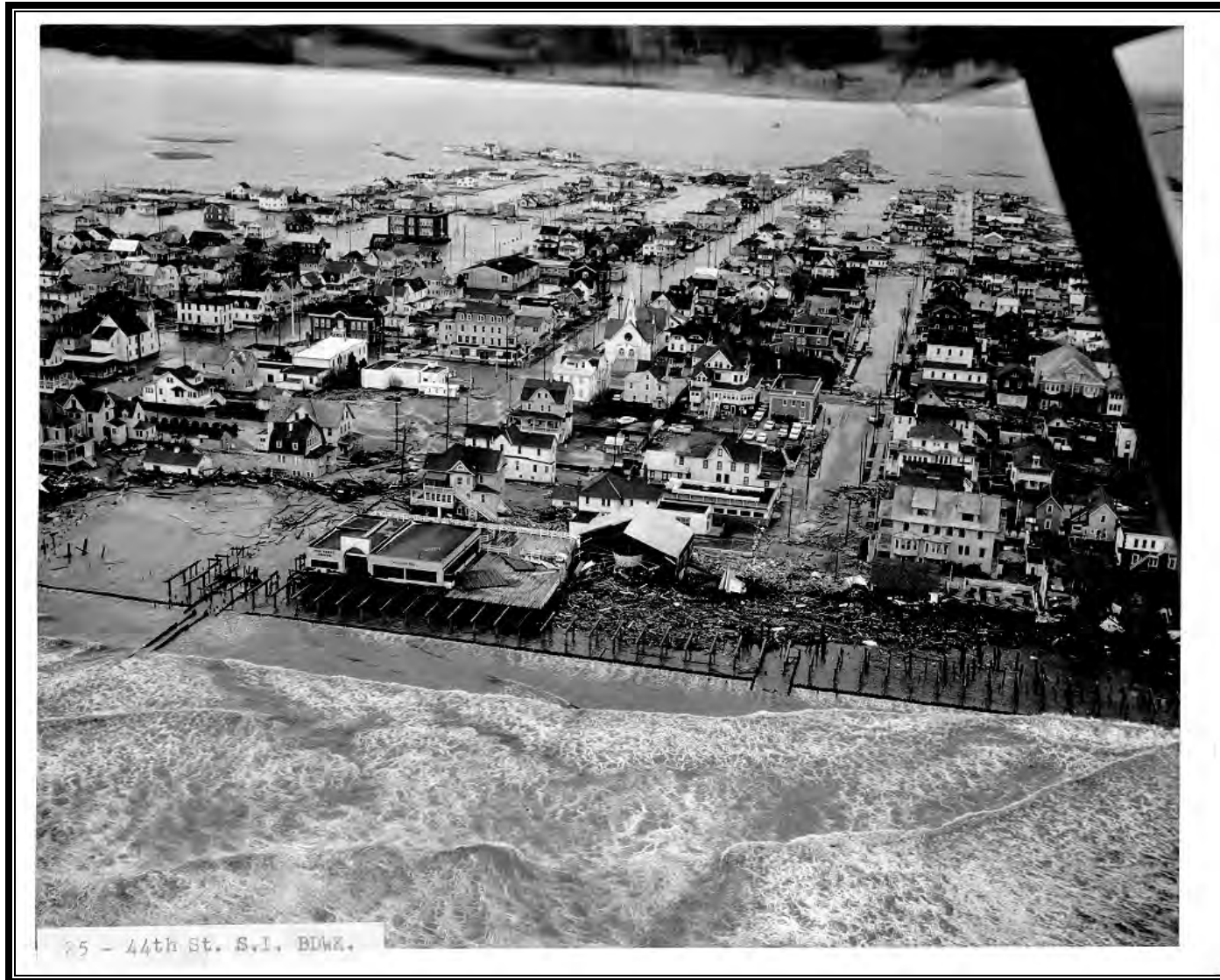
Photo 3-21 Sea Isle City (44 th Street), NJ. Storm of 1962.
