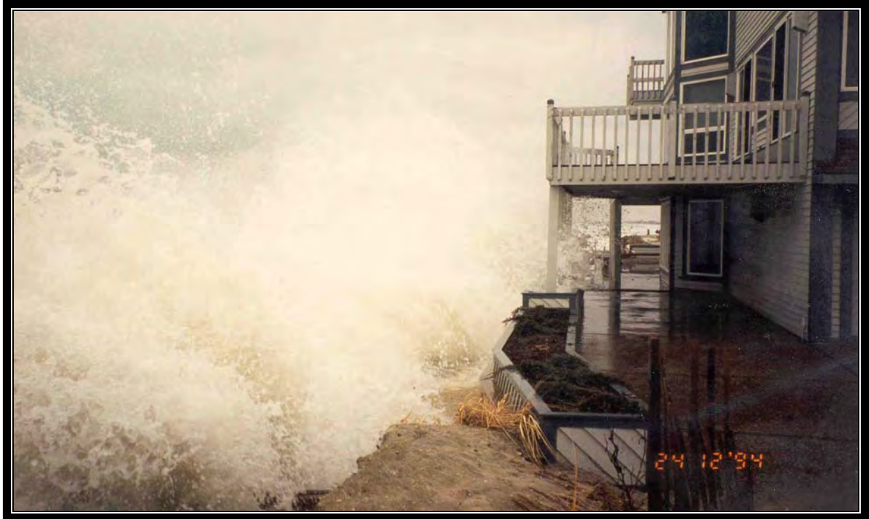
Photo 3-7 Strathmere, NJ - 12/24/94. Overtopping of bulkhead during minor storm event
