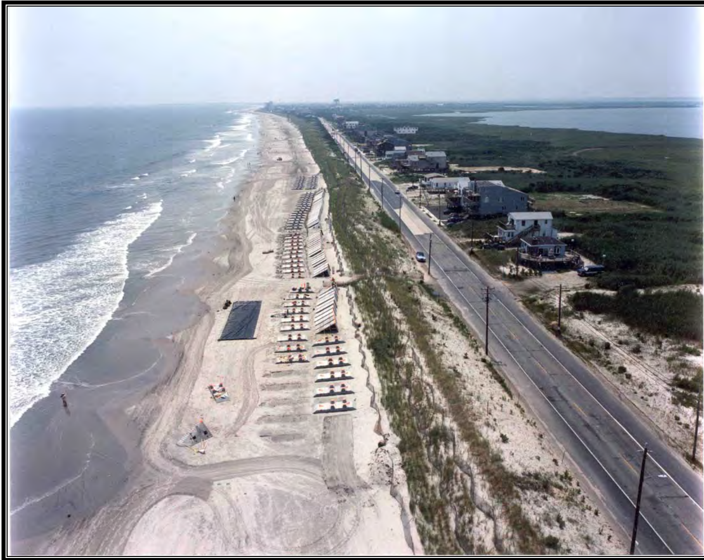
Photo 3-9 Whale Beach area, Sea Isle City, NJ - 7/25/89. Structures shown on beach were experimental shore protection devices, since removed.
