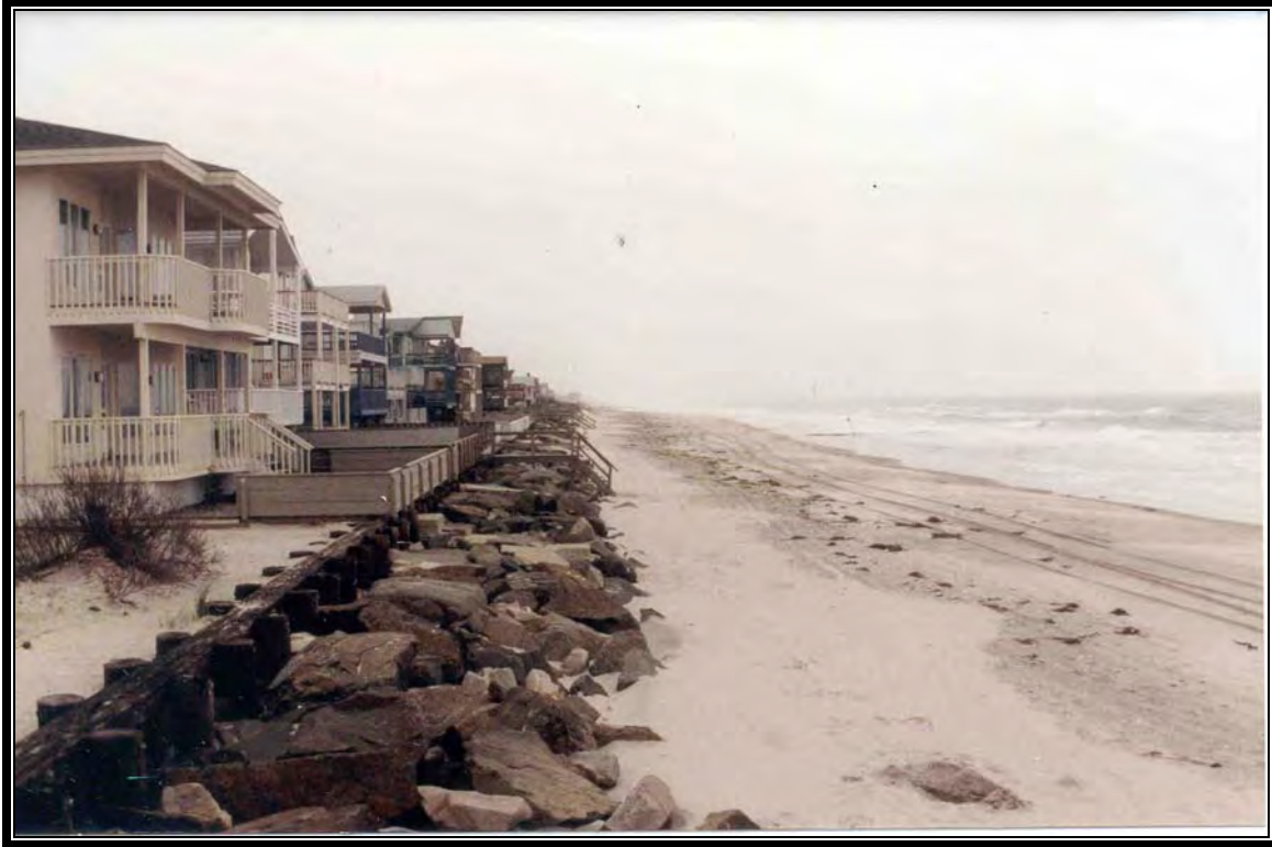
Photo 3-1 South End Ocean City, NJ (looking northeast). Note lack of dunes and proximity of high water line.
