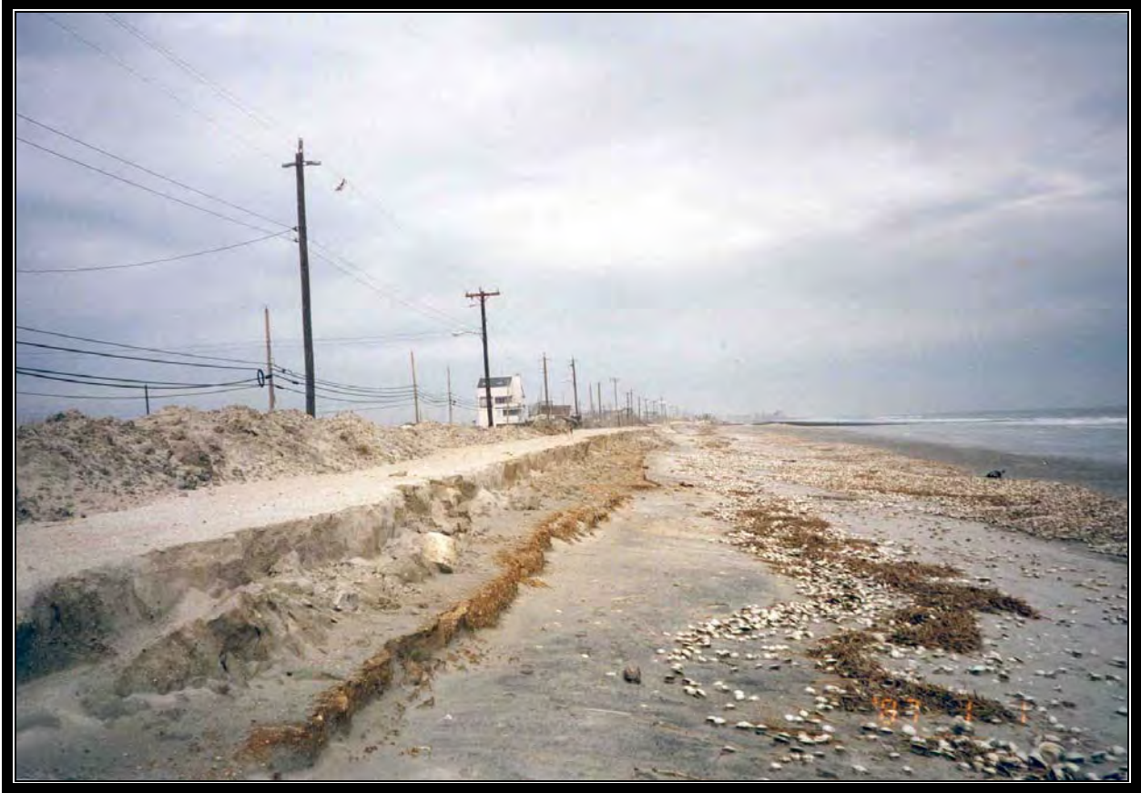
Photo 3-12 Whale Beach area, Sea Isle City, NJ - 2/96. FEMA-sponsored dunes eroded away by storms
