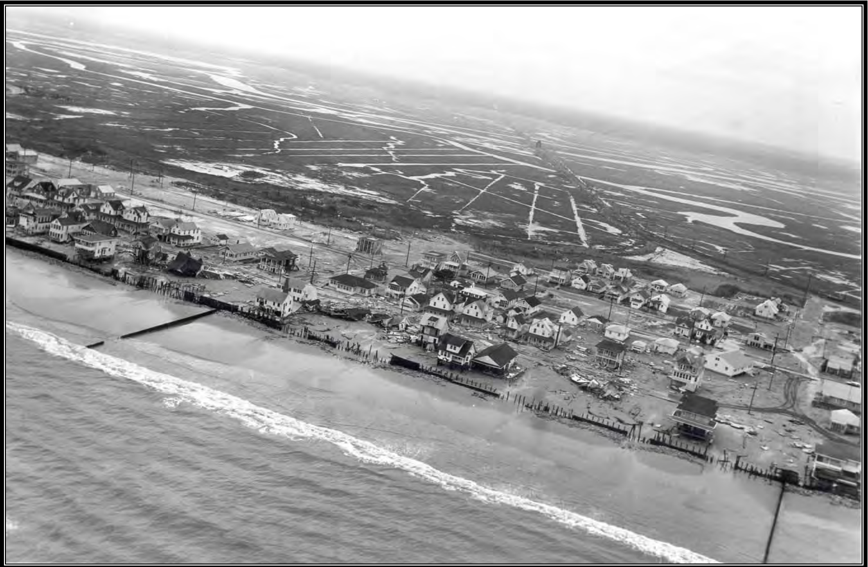
Photo 3-3 Ocean City, NJ (vic. 34 th Street). Storm of March 1962.
