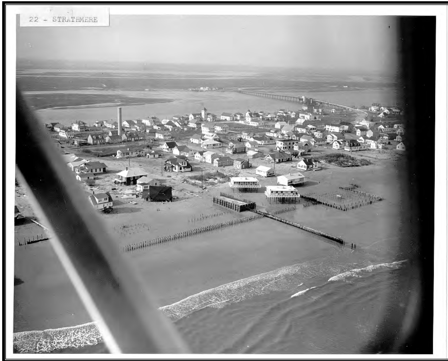
Photo 3-18 Strathmere, Upper Township, NJ. Storm of 1962.
