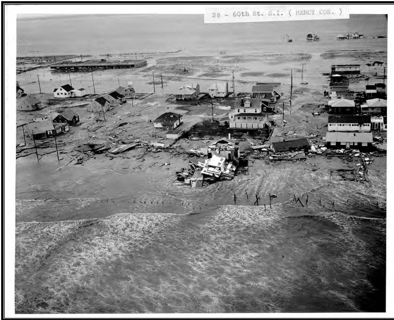
Photo 3-23 Sea Isle City (60 th Street), NJ. Storm of 1962.
