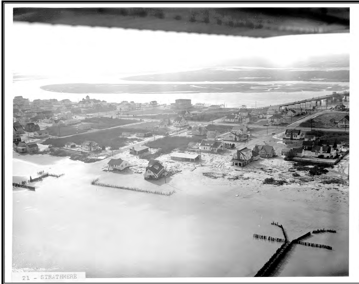
Photo 3-17 Strathmere, Upper Township, NJ. Storm of 1962.
