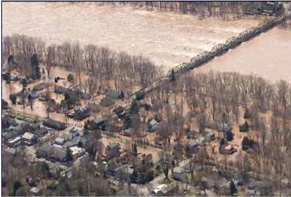
Flooding in the Study Area, April 2005
