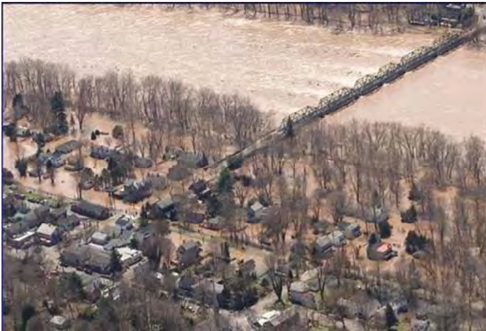
Flooding in the Study Area, April 2005
