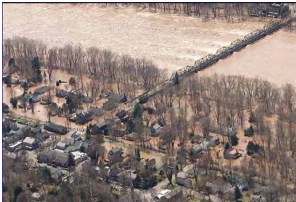
Flooding in the Study Area, April 2005
