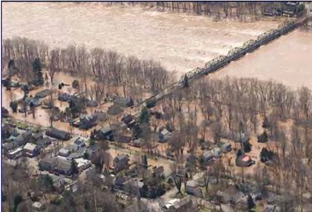
Flooding in the Study Area, April 2005
