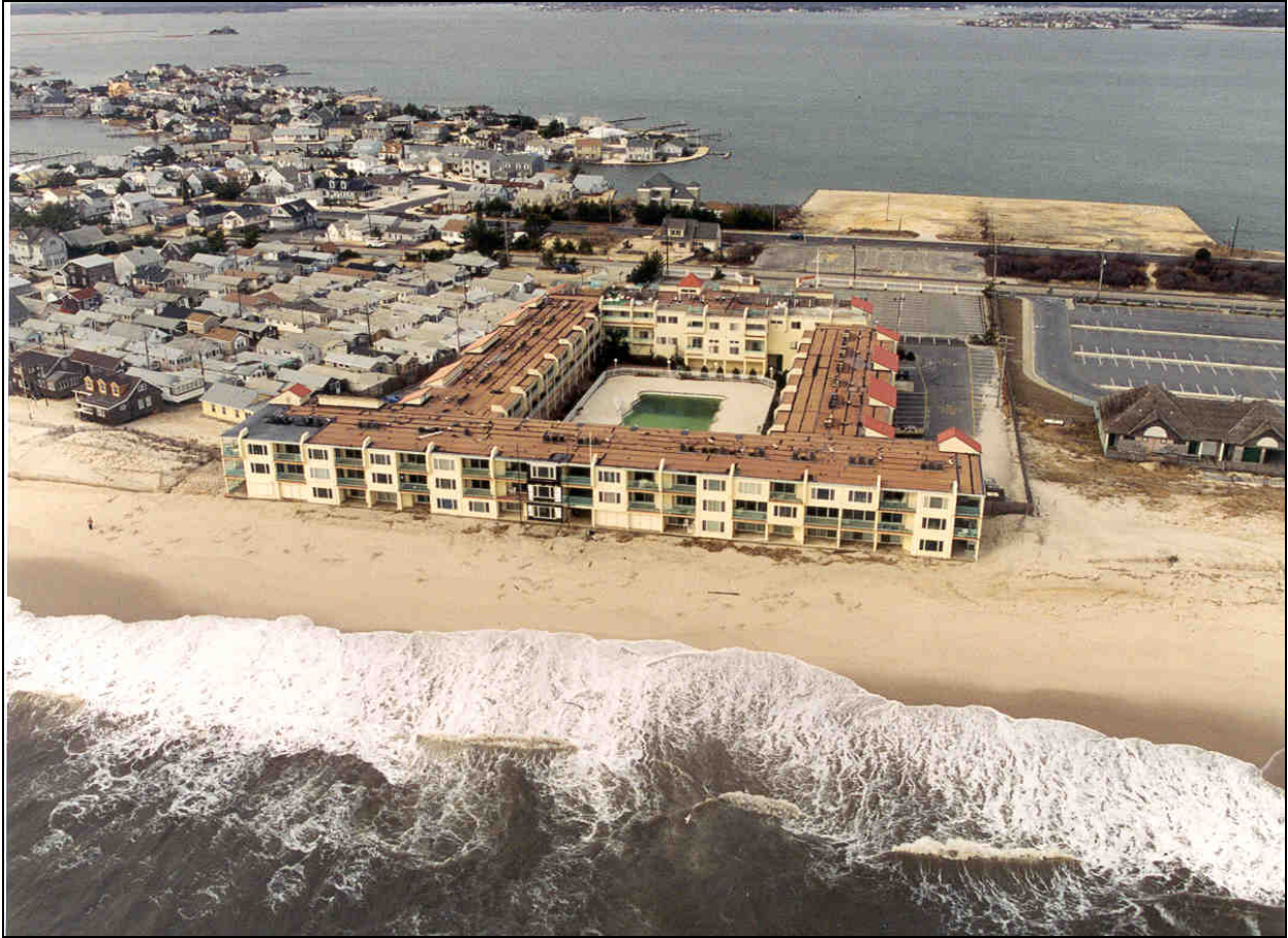
Figure 1-7 Brick Township, NJ - 02/06/98
