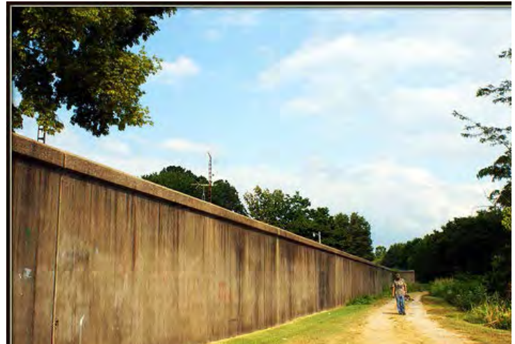
Brookport, IL Floodwall
