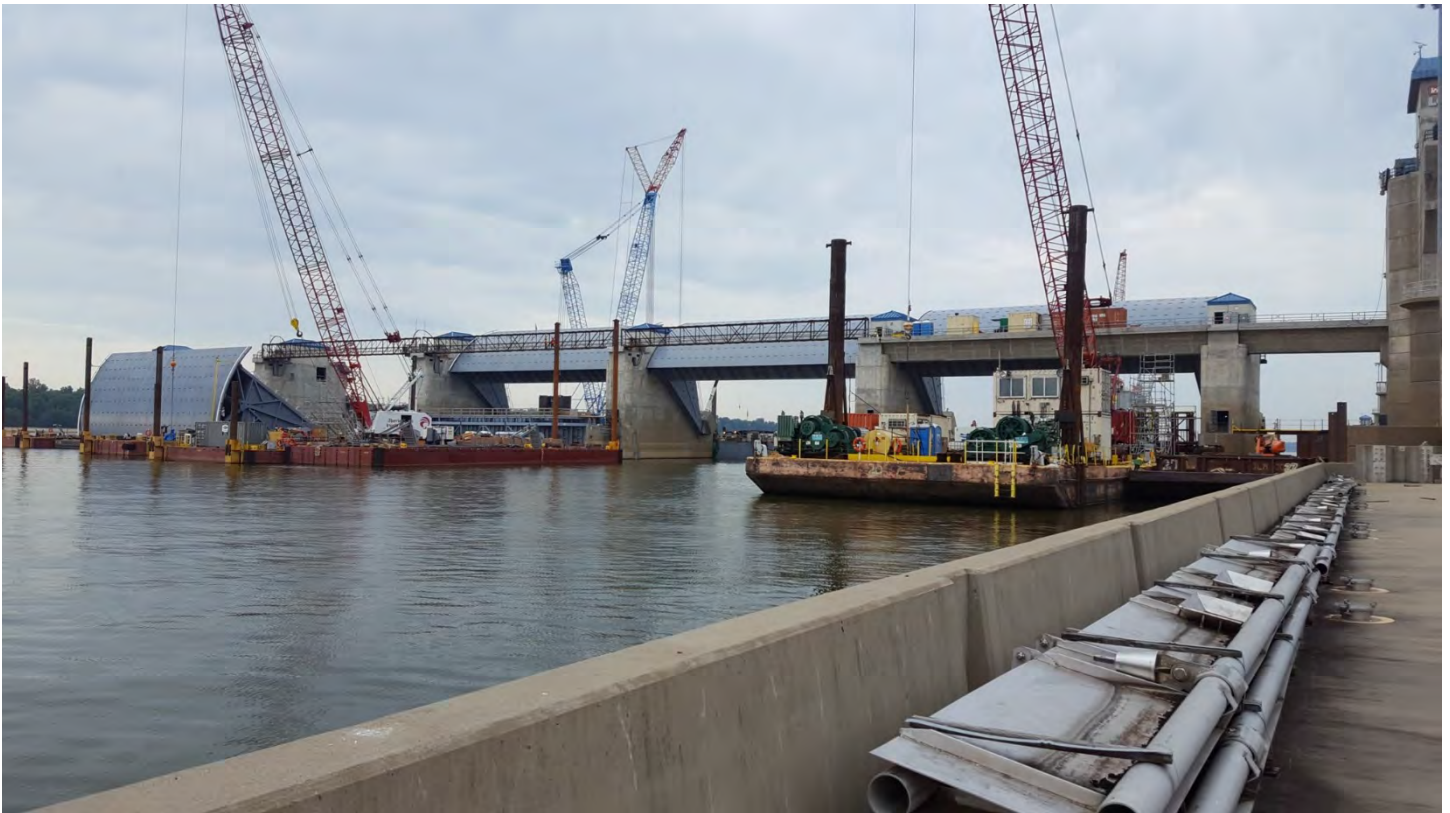
Tainter Gates #1, #2 and #3 erected. Tainter Gate #4 delivered (far left).
