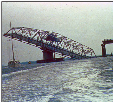
The Ben Sawyer Bridge to Sullivan's Island, SC, was damaged by Hurricane Hugo in 1989. Photo credit NOAA/National Weather Service
