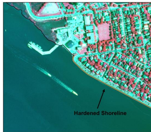
Figure 1.3.5. Hardened Shoreline, seawall, rip-rap
