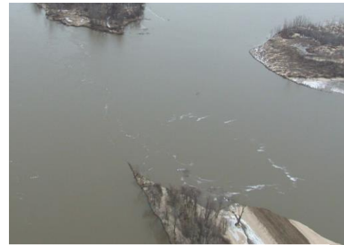
Critical bankline failures from winter flooding repaired under emergency
