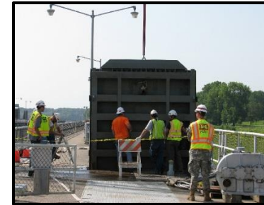
Bulkhead is inspected prior to culvert valve inspection.
