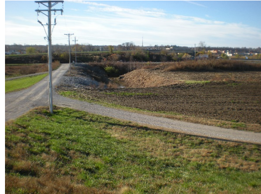
Watershed 4 Pump Station Site.
