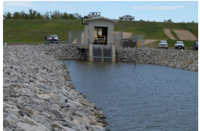
Missouri Chute Pump Station
